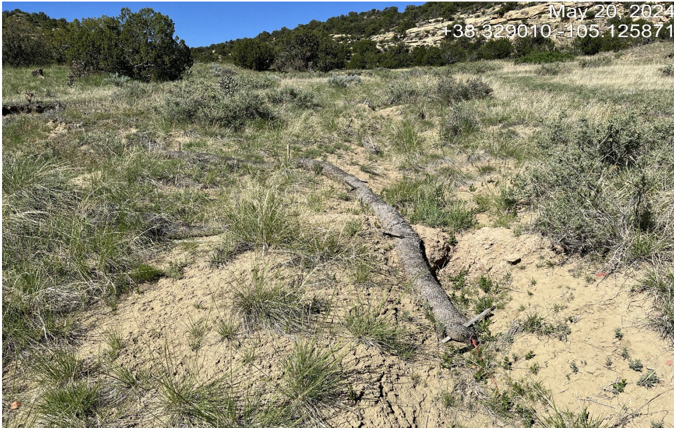
Photo 5. Facing southwest along the former access road. It appears that the stormwater from the location is directed down the road which is causing erosion issues shown in previous photos. Wattles that were installed have been washed out.
