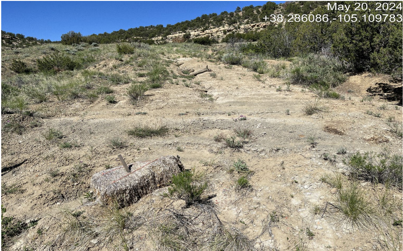
Photo 1. Facing southwest toward the former access road. This area is not stabilized with vegetation and there is erosion has occurred. It appears topsoil has been scoured off this area of the former road. Previous corrective action was not completed.
