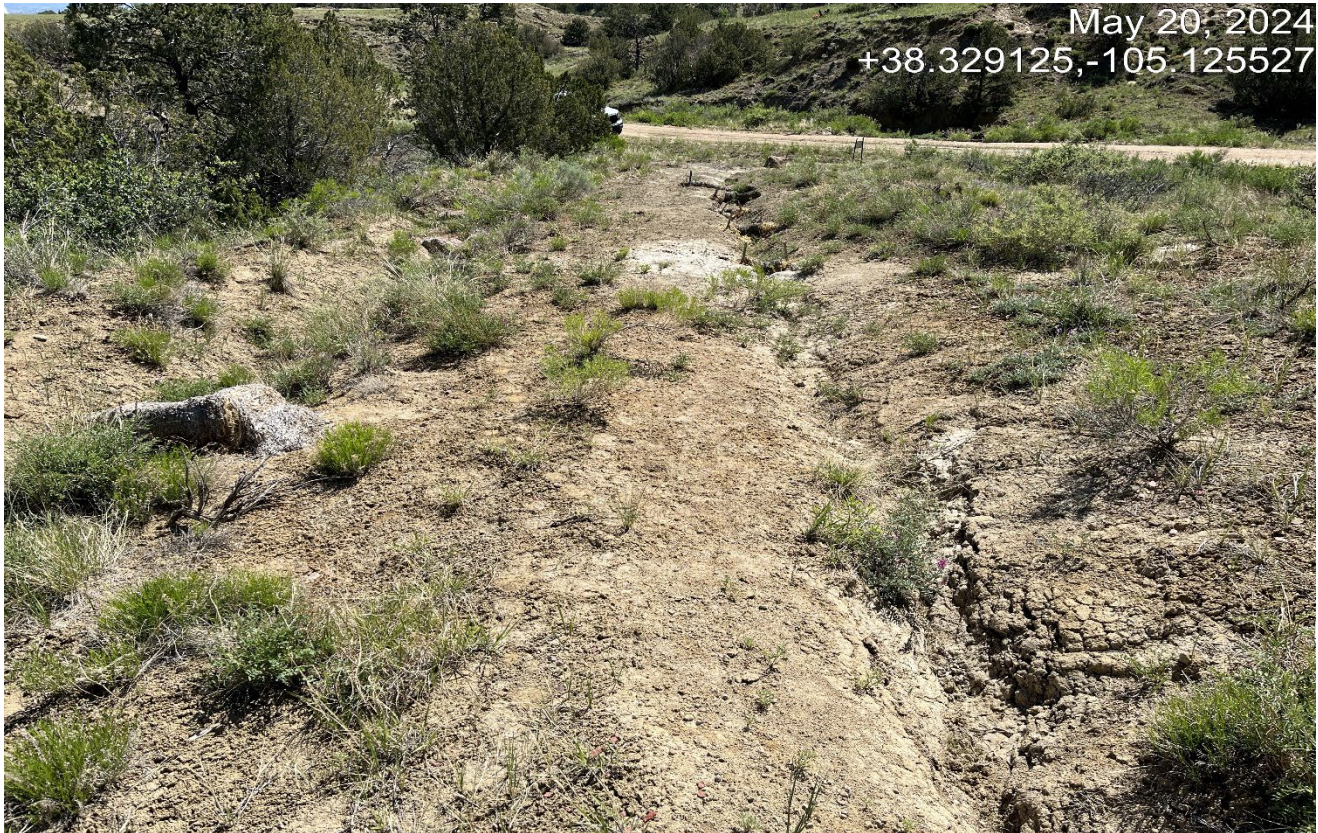
Photo 3. Facing back down the access road. There is stormwater erosion occurring on both side of the former road. Straw bales were placed on the left side and not staked in. The bales are degrading and are insufficient. This area needs to be reclaimed and stabilized for long term stabilization.
