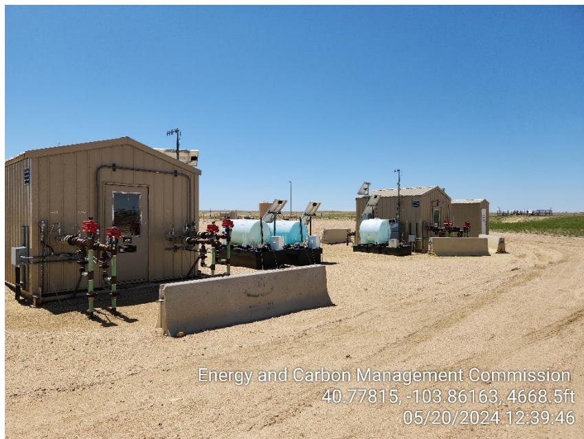
Photo 1 – Gas Lift Injection Meter Houses
