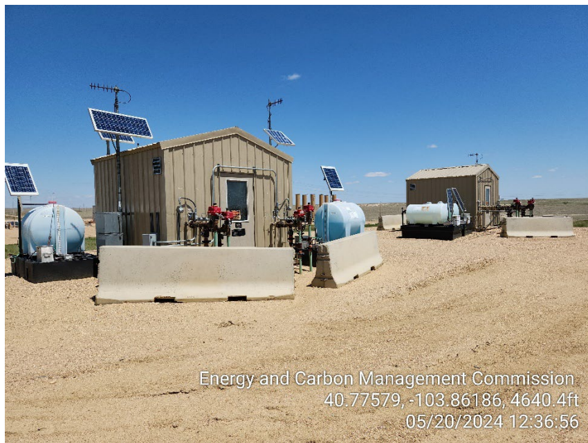
Photo 1 – Gas Lift Injection Meter Houses
