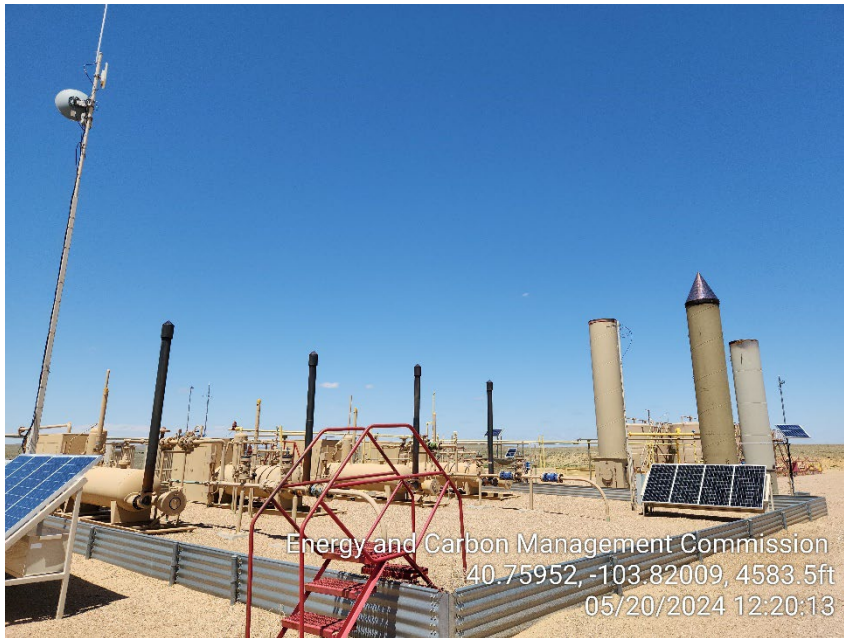
Photo 5 – Separators and ECDs
