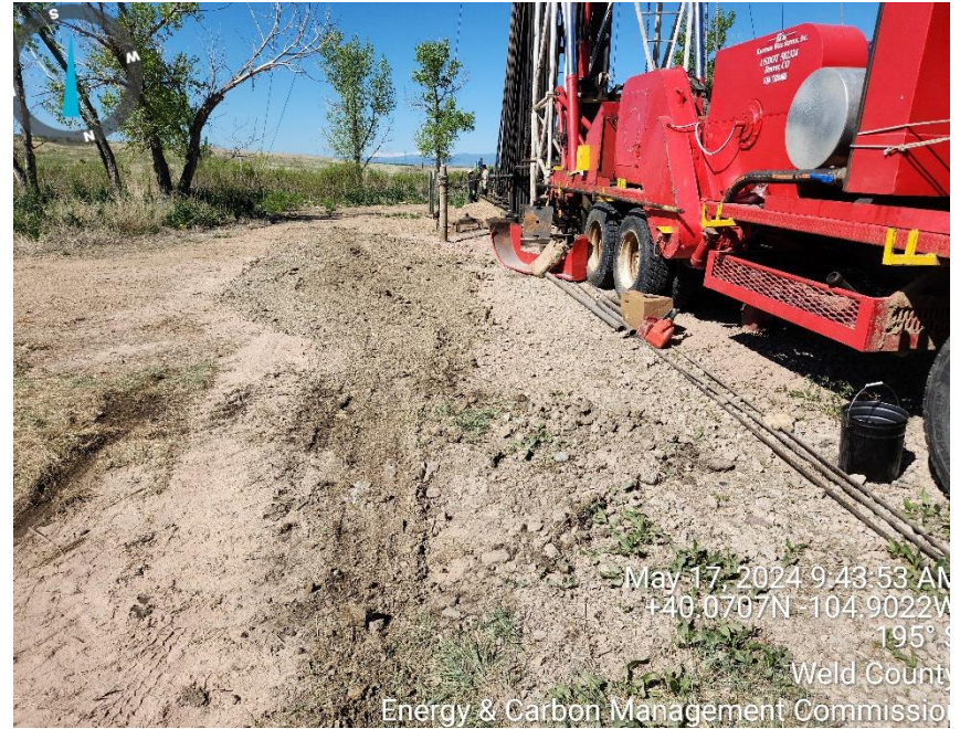
Photo 4 rig 7 and equipment
