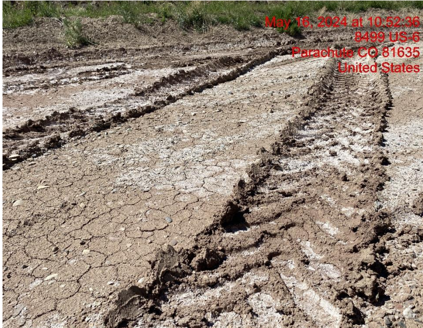
Lack of Stabilization – Photo #01251
