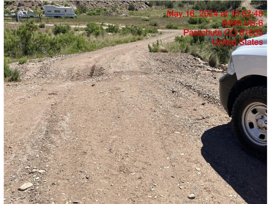
Insufficient Vehicle Tracking BMPs at Location Entrance/Exit – Photo #01252
