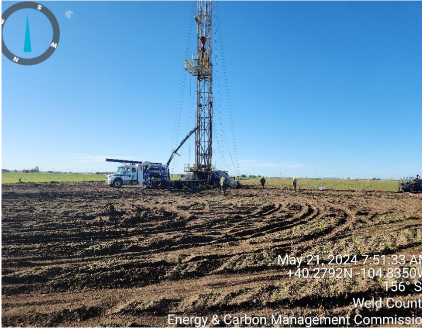
Photo 3 rig 351, wire line unit and equipment
