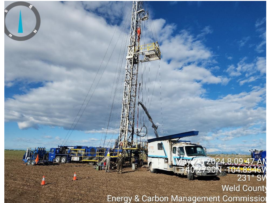
Photo 6 rig 351, wire line unit and equipment
