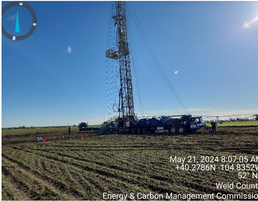
Photo 5 rig 351 and equipment
