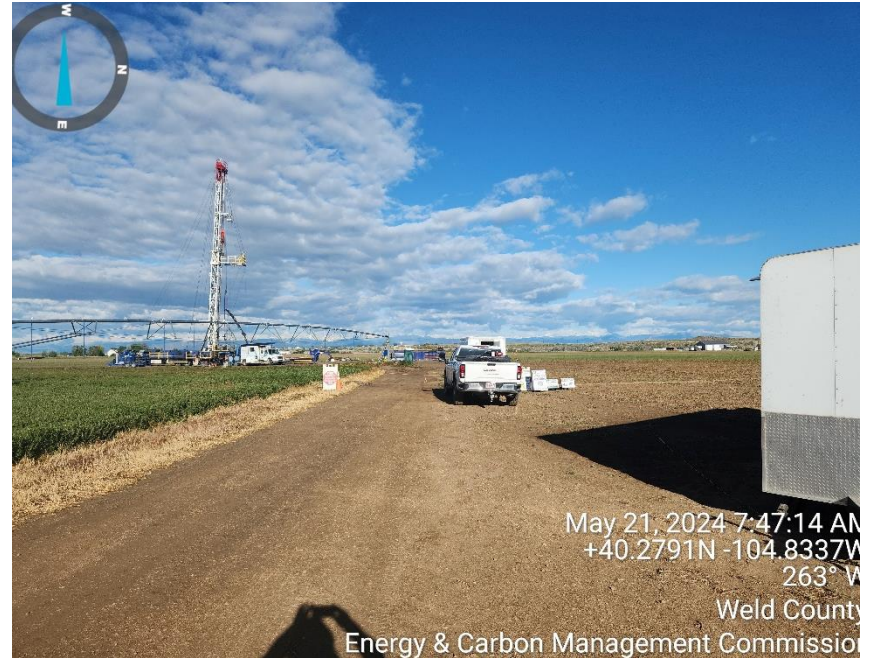
Photo 2 entrance to site
