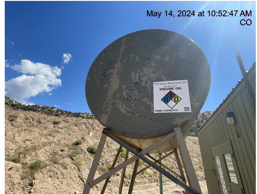
Photo # 6941 Capacity on tank label faded & becoming illegible
