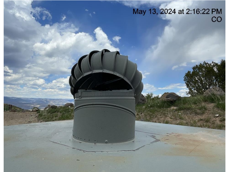
Photo # 6806 Turbine not properly installed on unused equipment/wildlife hazard/available for entry by wildlife
