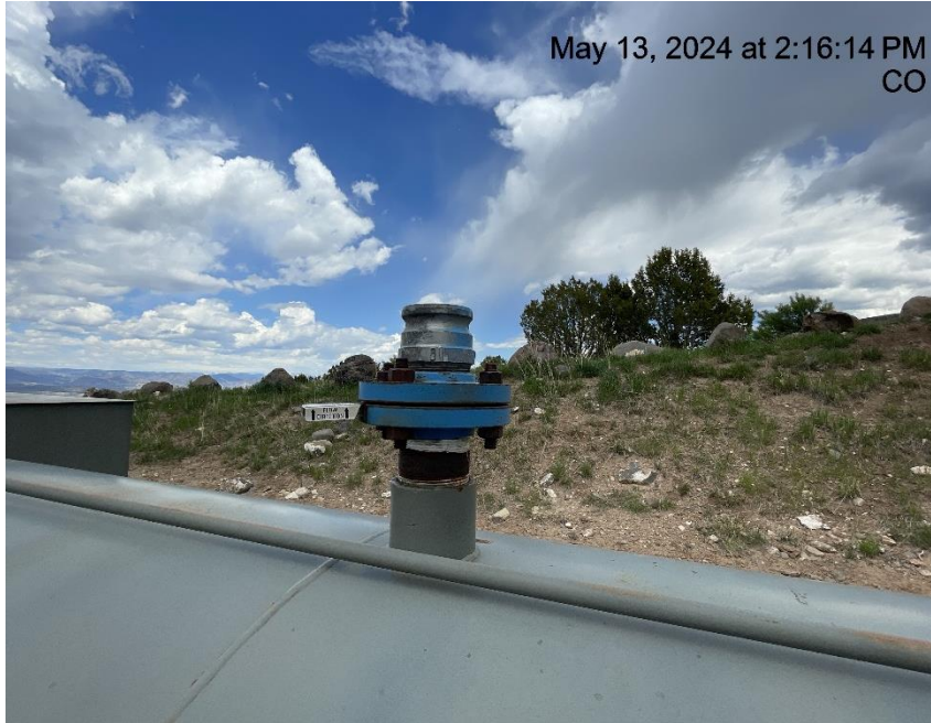
Photo # 6805 Open ended piping on unused equipment /wildlife hazard/available for entry by wildlife
