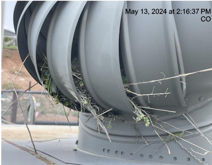
Photo # 6807 Possible nest inside turbine on unused equipment
