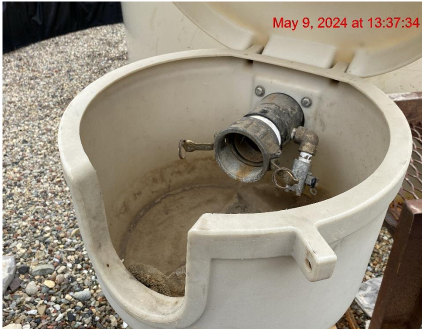
Open-Ended Load Line – Photo #01108
