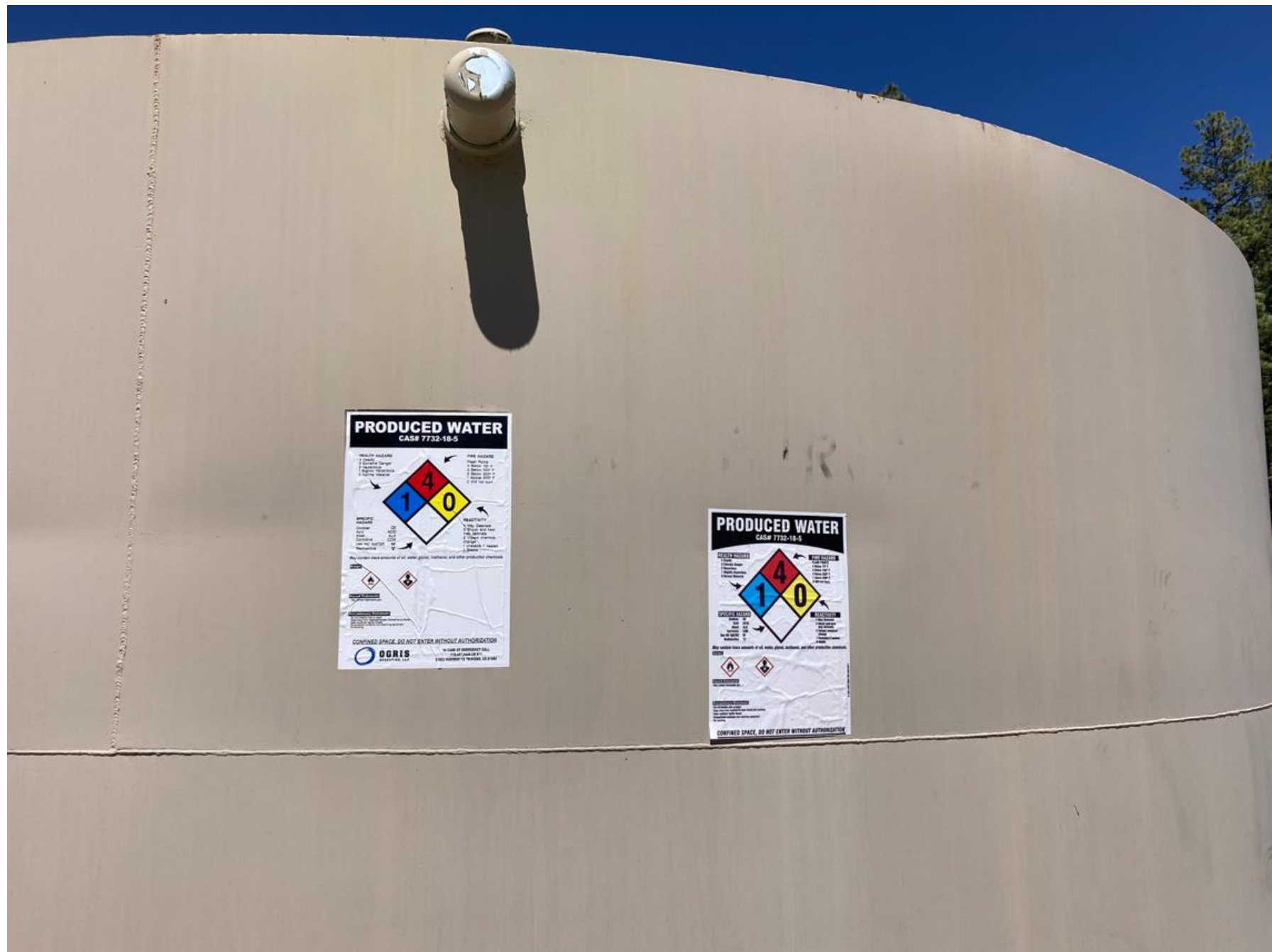
PHOTO 2: THE NFPA STICKERS HAVE BEEN REPLACED, SHOWING CORRECT OPERATOR NAME AND CONTACT NUMBER.
