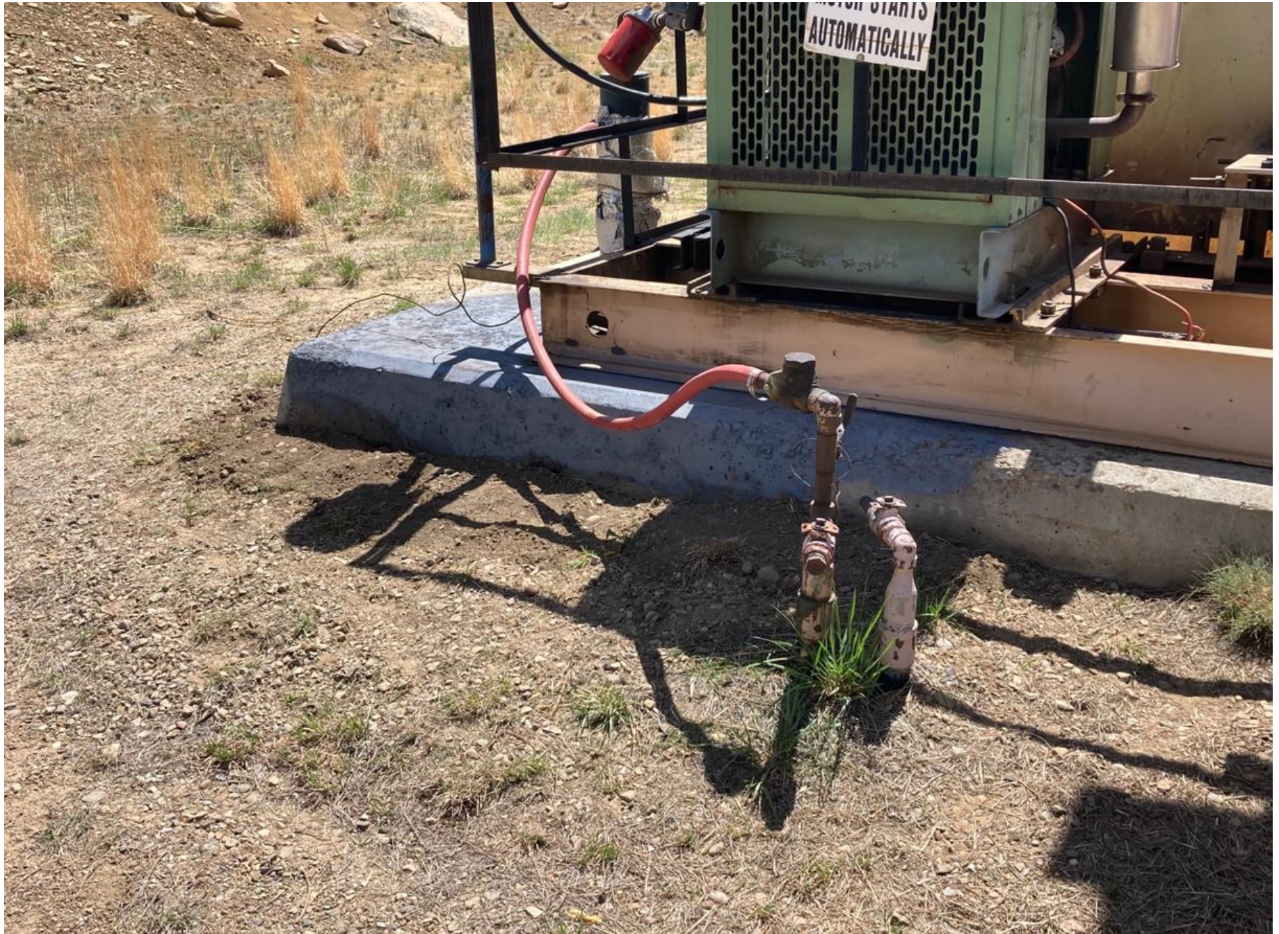
PHOTO 1: THE SOIL STAINS HAVE BEEN REMOVED, THE CONCRETE RISER HAS BEEN PAINTED, AND THE PUMPING UNIT SKID HAS BEEN CLEANED. MAINTENANCE HAS BEEN PERFORMED TO ALL EQUIPMENT AND THE SELF INSPECTION PROCESS HAS BEEN REVIEWED.
