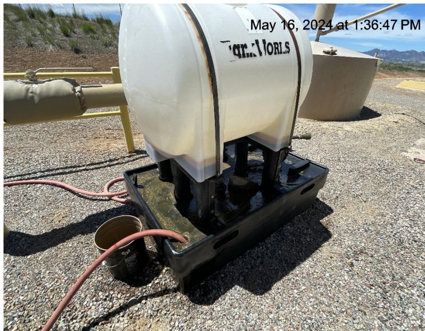
Photo # 7437 Chemical tank containment evacuated of fluids by TEP employee
