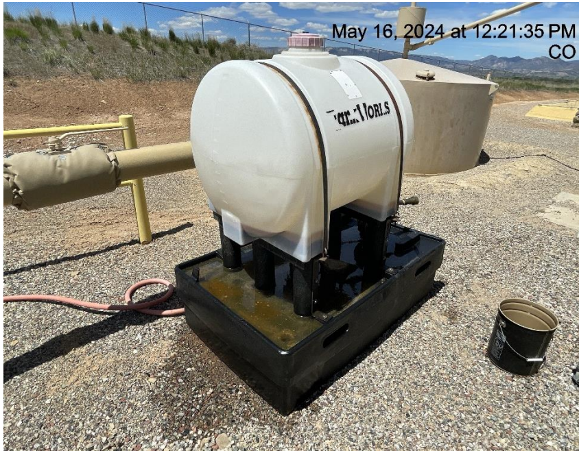
Photo # 7435 Failure to maintain chemical BMP - Chemical tank containment full of fluid/fluid overflowed containment & spilled on the ground
