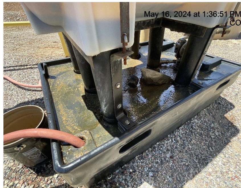
Photo # 7438 Chemical tank containment evacuated of fluids by TEP employee
