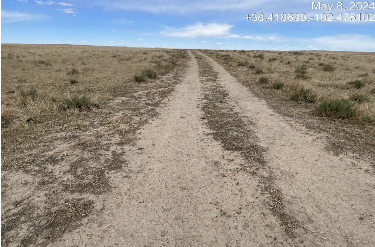
Photo 1. Facing north toward the access road which is not establishing vegetation. It does not appear reclamation was completed.
