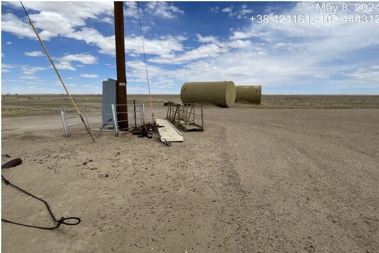
Photo 5. Facing east. There are two steel tanks that are unused that need to be removed along with various parts by the power pole.
