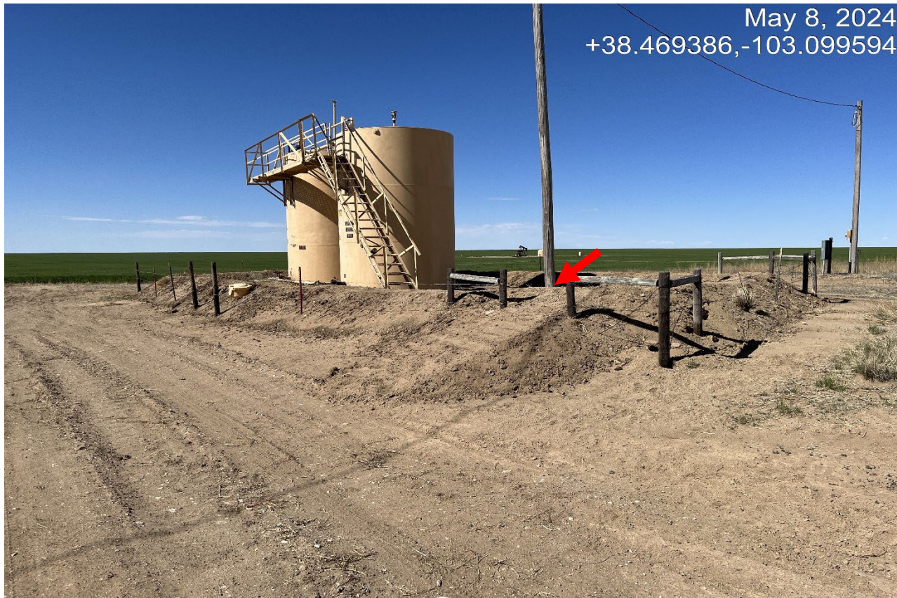
Photo 1. Facing toward the offsite tank battery location. It appears some work has started at the tank battery but is incomplete. No sign has been installed. The fence is not adequate to prevent livestock entry and there is no gate at the red arrow.
