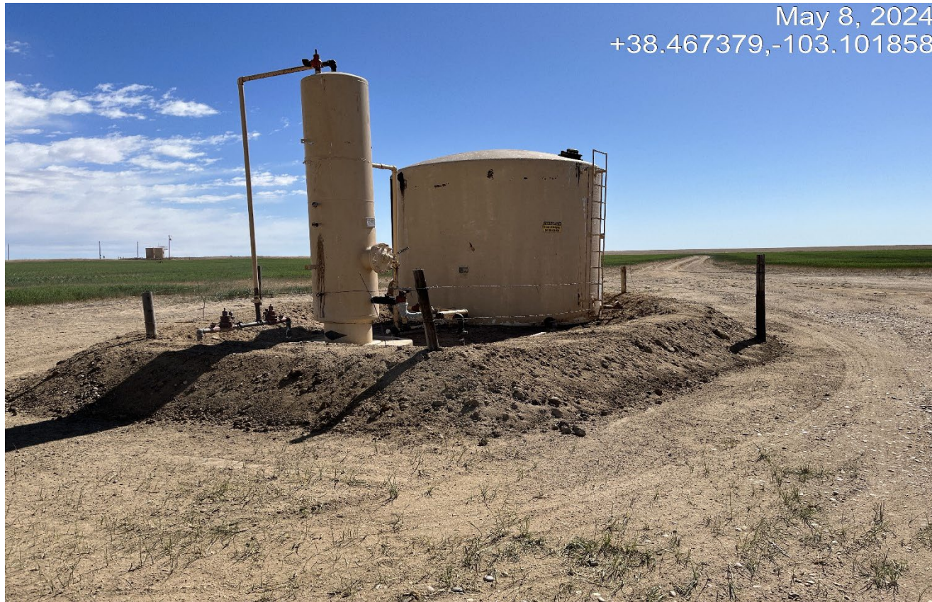
Photo 3. Facing toward the tank. The berm around the tank has been rebuilt. The sides of the berm are not compacted.
