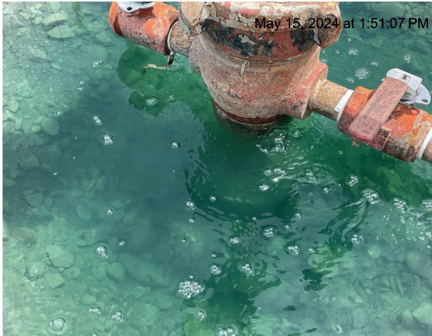
Photo # 7061 Possible wellhead leak on W 15-5 well
