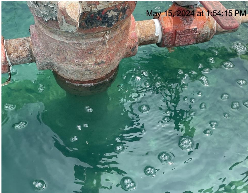
Photo # 7063 Possible wellhead leak on W 15-5 well
