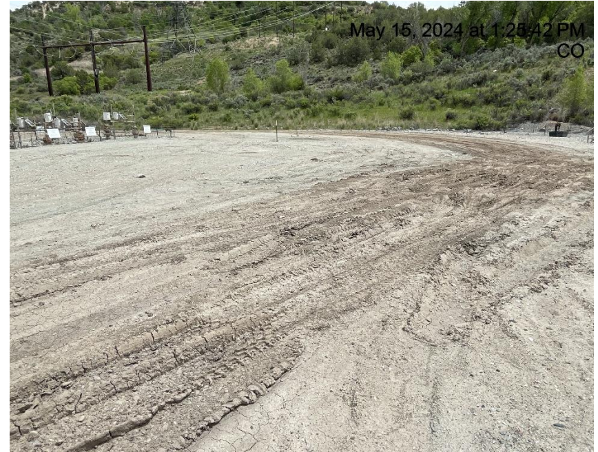
Photo # 7086 Lack of stabilization/compaction/insufficient BMP's
