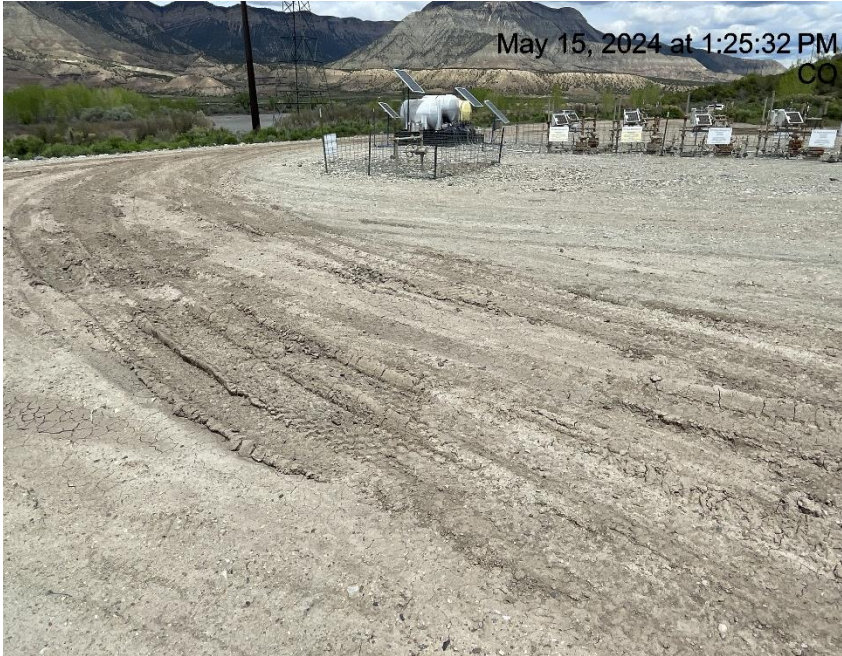
Photo # 7085 Lack of stabilization/compaction/insufficient BMP's
