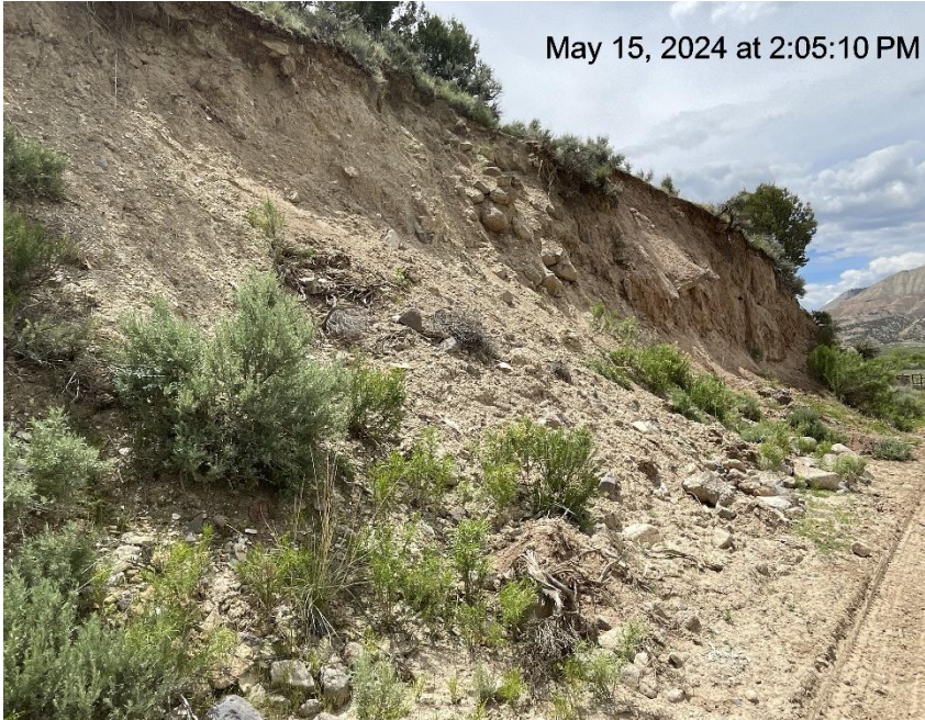
Photo # 7099 Lack of stabilization & erosion on cut slope /insufficient BMP's
