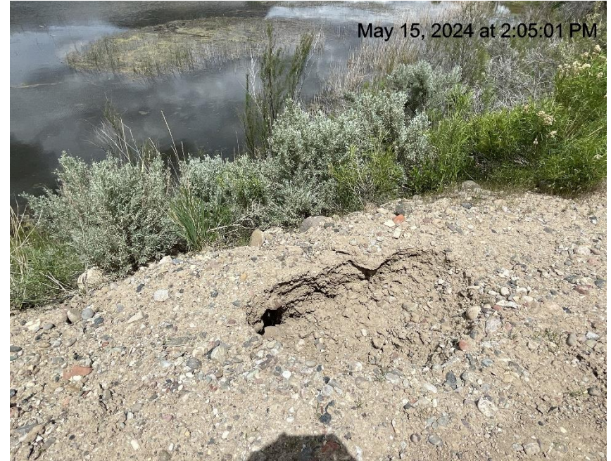
Photo # 7102 Tunnel erosion on lease road (approximately 6/10th of a mile from location)
