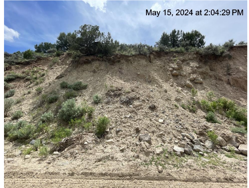
Photo # 7098 Lack of stabilization & erosion on cut slope /insufficient BMP's
