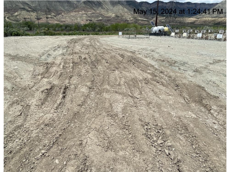
Photo # 7080 Lack of stabilization/compaction/insufficient BMP's
