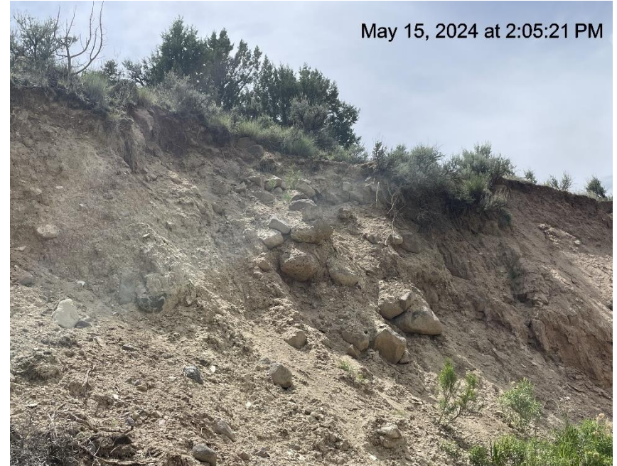
Photo # 7100 Lack of stabilization & erosion on cut slope /insufficient BMP's
