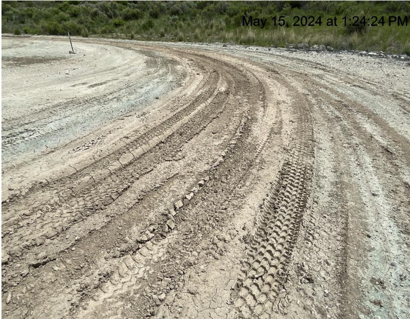
Photo # 7079 Lack of stabilization/compaction/insufficient BMP's
