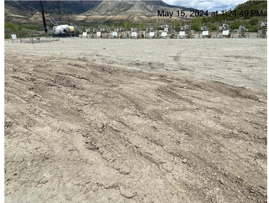
Photo # 7082 Lack of stabilization/compaction/insufficient BMP's
