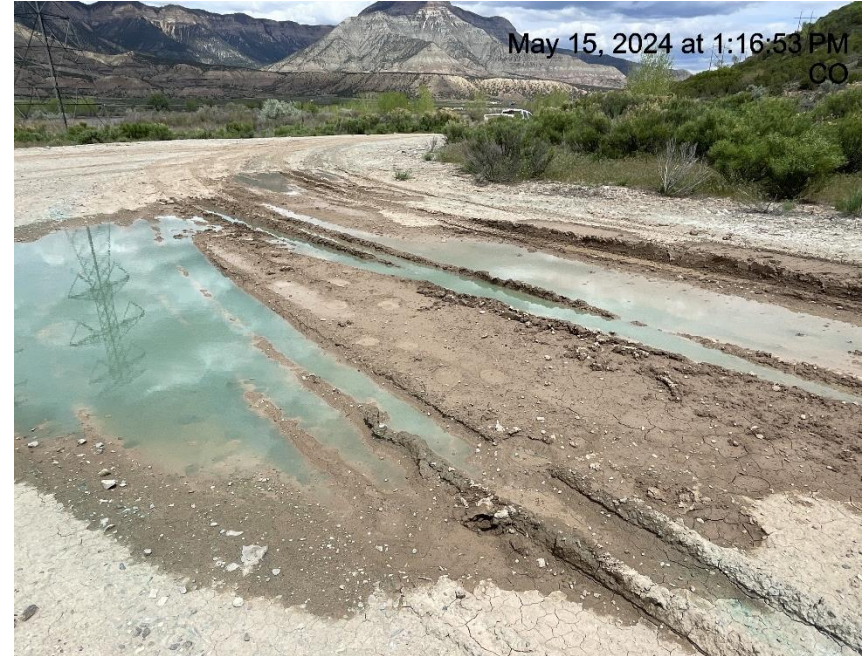
Photo # 7074 Location surface lacks stabilization/compaction with insufficient vehicle tracking BMPs in place to minimize transportation of sediment
