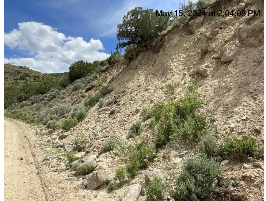
Photo # 7096 Lack of stabilization & erosion on cut slope /insufficient BMP's
