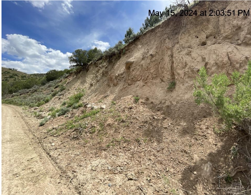
Photo # 7093 Lack of stabilization & erosion on cut slope /insufficient BMP's
