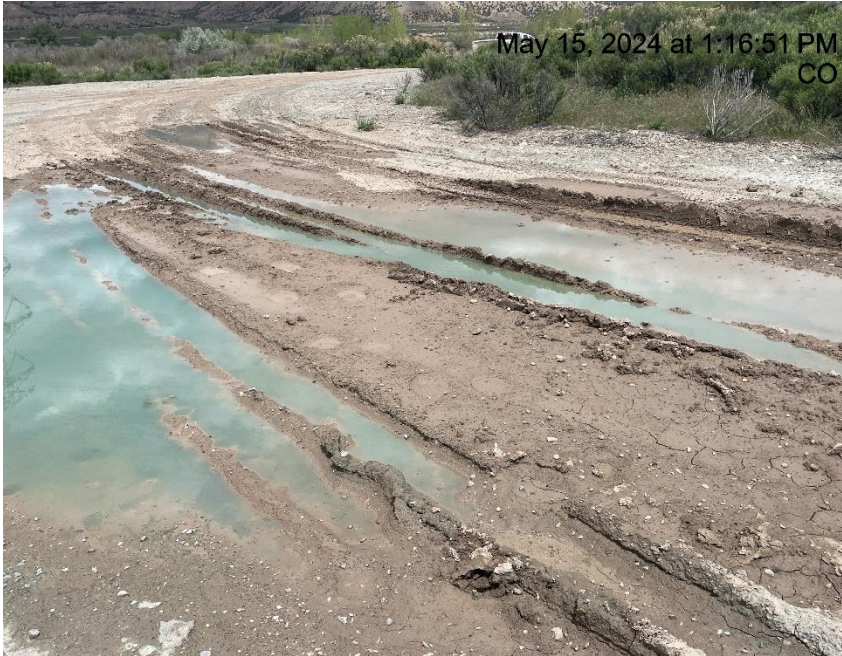
Photo # 7073 Location surface lacks stabilization/compaction with insufficient vehicle tracking BMPs in place to minimize transportation of sediment
