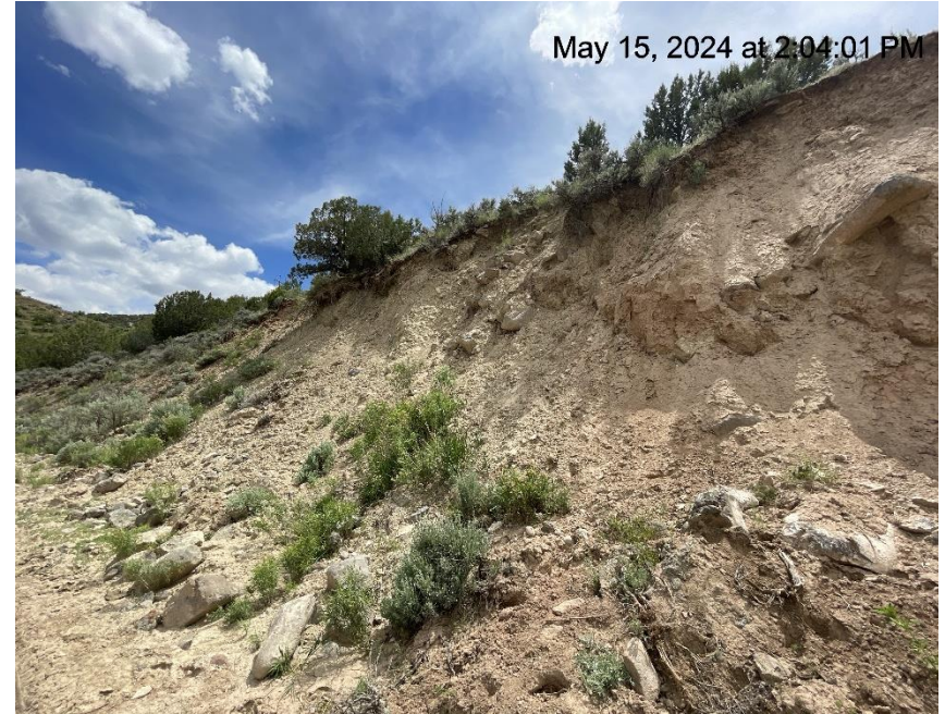
Photo # 7094 Lack of stabilization & erosion on cut slope /insufficient BMP's
