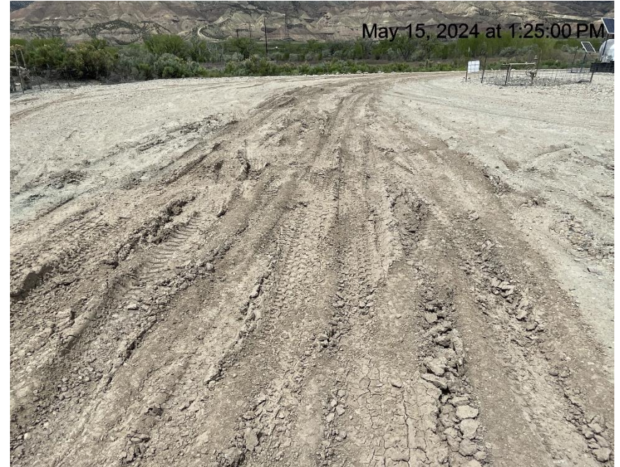
Photo # 7084 Lack of stabilization/compaction/insufficient BMP's
