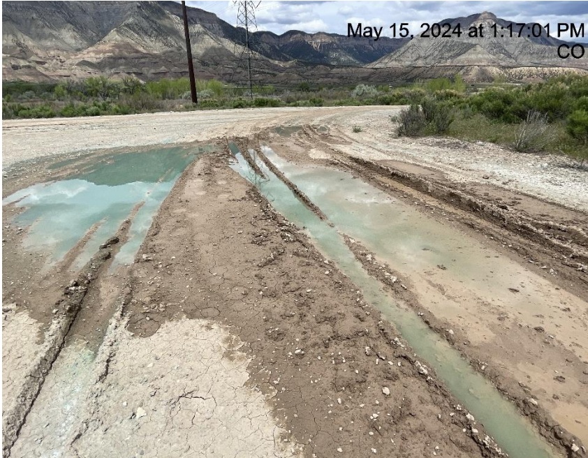
Photo # 7075 Location surface lacks stabilization/compaction with insufficient vehicle tracking BMPs in place to minimize transportation of sediment
