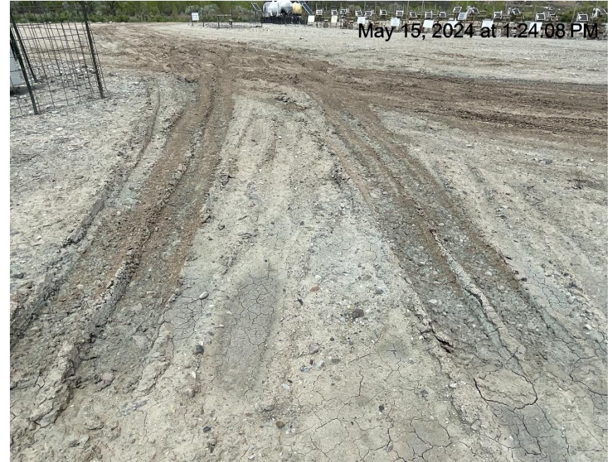
Photo # 7078 Lack of stabilization/compaction/insufficient BMP's
