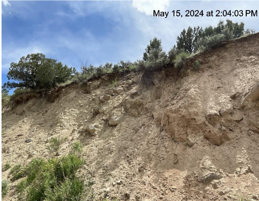
Photo # 7095 Lack of stabilization & erosion on cut slope /insufficient BMP's
