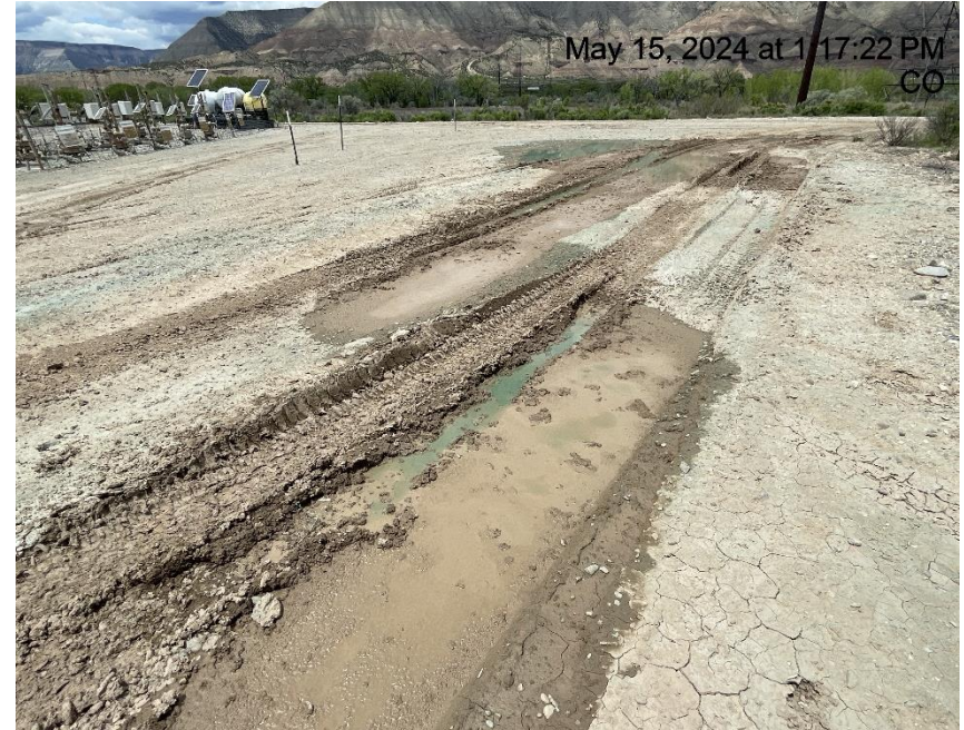
Photo # 7076 Lack of stabilization/compaction/insufficient BMP's
