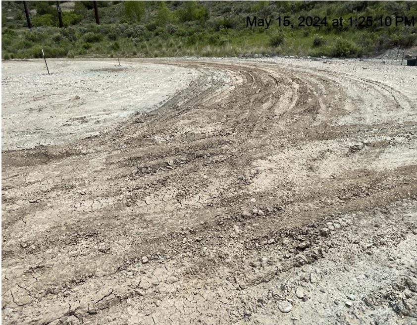
Photo # 7083 Lack of stabilization/compaction/insufficient BMP's
