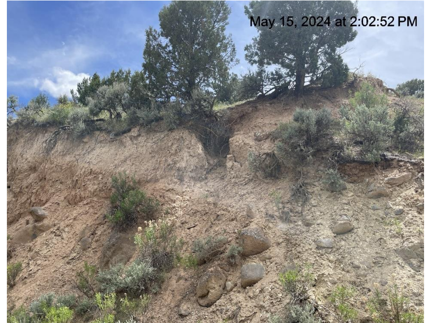
Photo # 7088 Lack of stabilization & erosion on cut slope /insufficient BMP's
