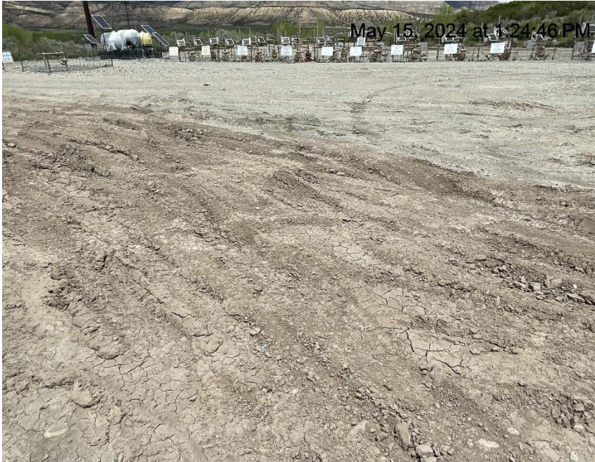
Photo # 7081 Lack of stabilization/compaction/insufficient BMP's
