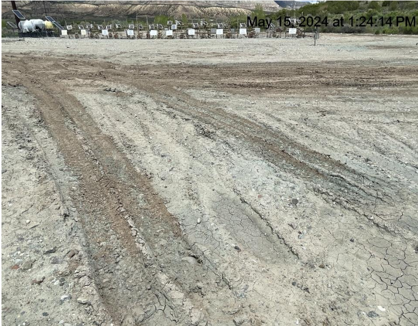
Photo # 7077 Lack of stabilization/compaction/insufficient BMP's
