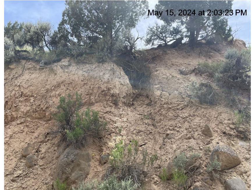
Photo # 7092 Lack of stabilization & erosion on cut slope /insufficient BMP's
