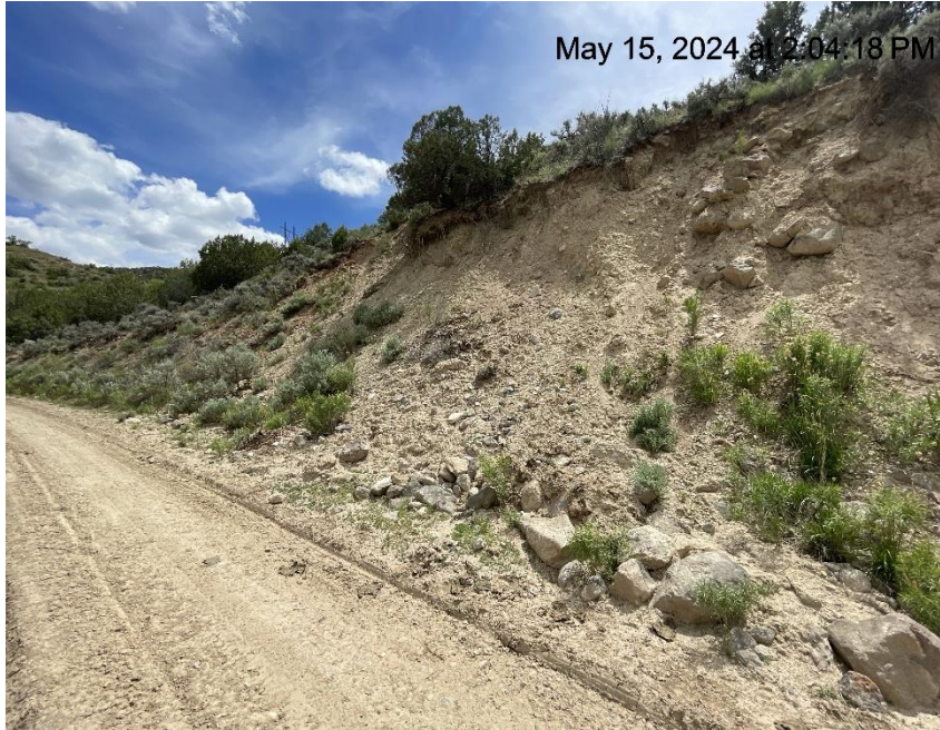
Photo # 7097 Lack of stabilization & erosion on cut slope /insufficient BMP's
