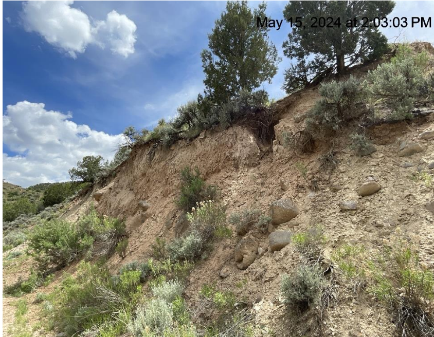
Photo # 7089 Lack of stabilization & erosion on cut slope /insufficient BMP's
