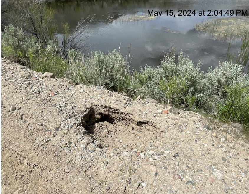
Photo # 7101 Tunnel erosion on lease road (approximately 6/10th of a mile from location)
