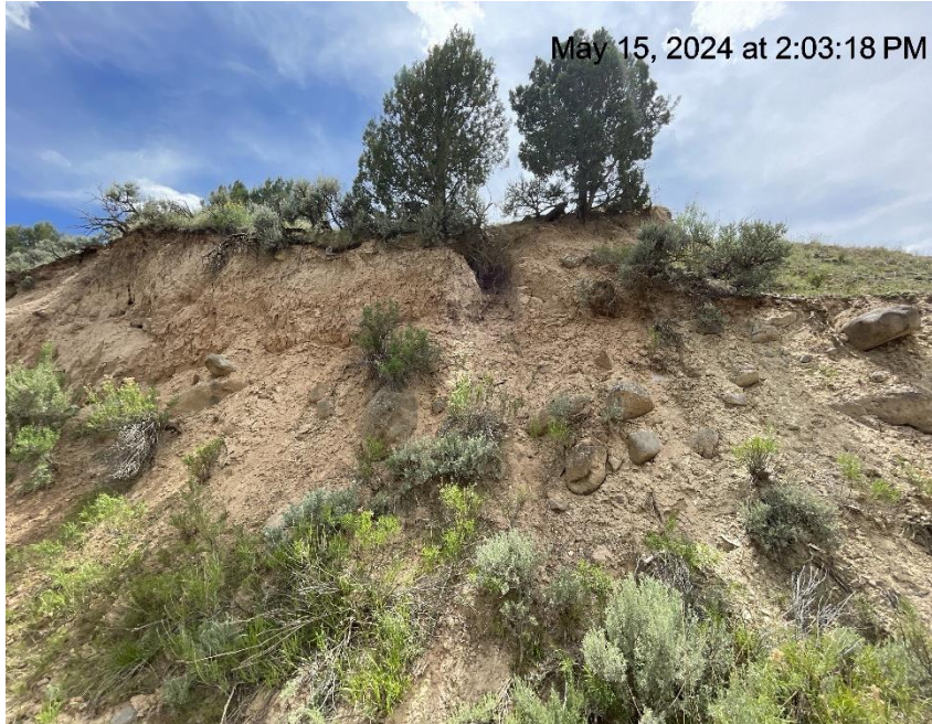
Photo # 7091 Lack of stabilization & erosion on cut slope /insufficient BMP's
