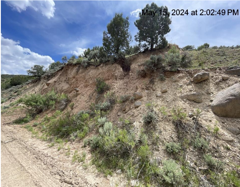
Photo # 7087 Lack of stabilization & erosion on cut slope /insufficient BMP's
