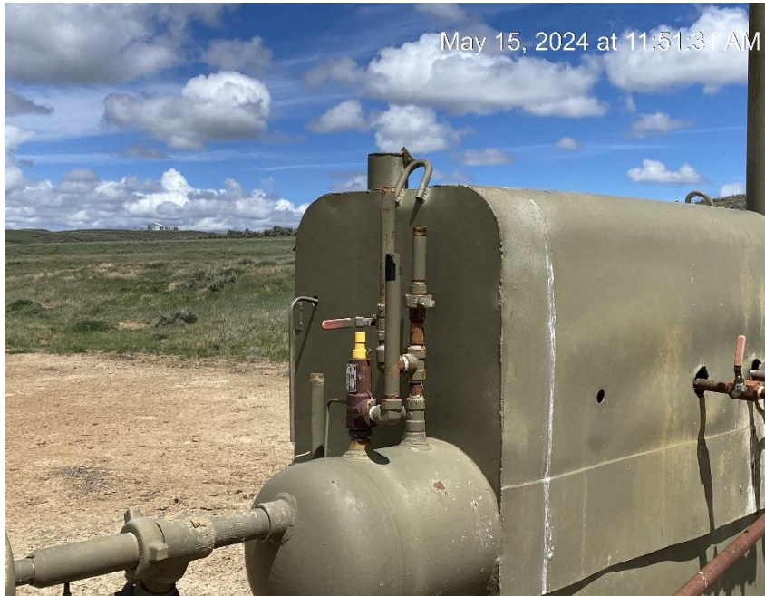
Relief risers missing protective caps
