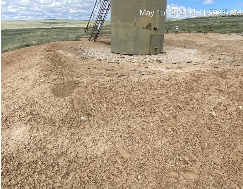
Tank berm needs maintenance
