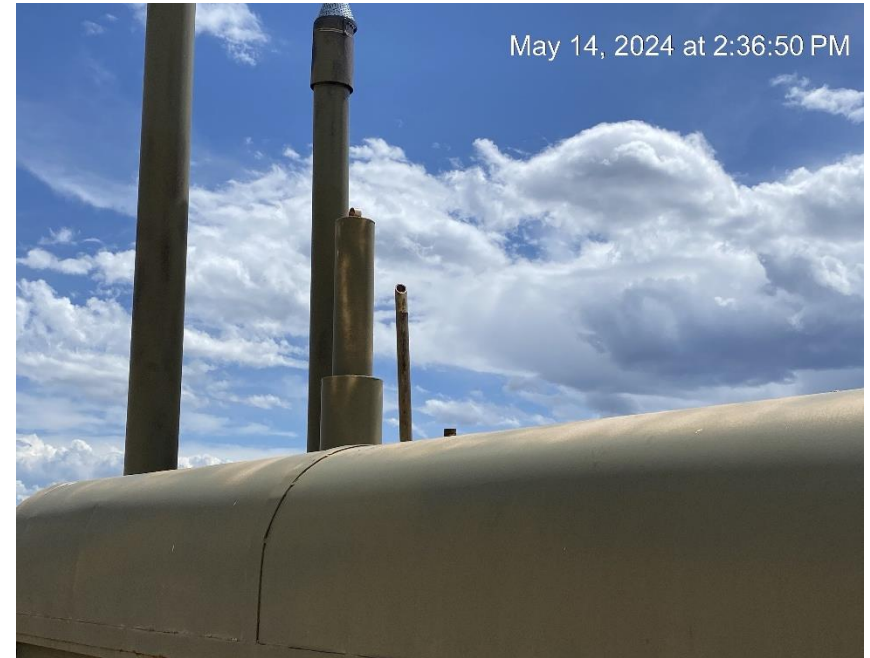
Missing cap on relief riser
