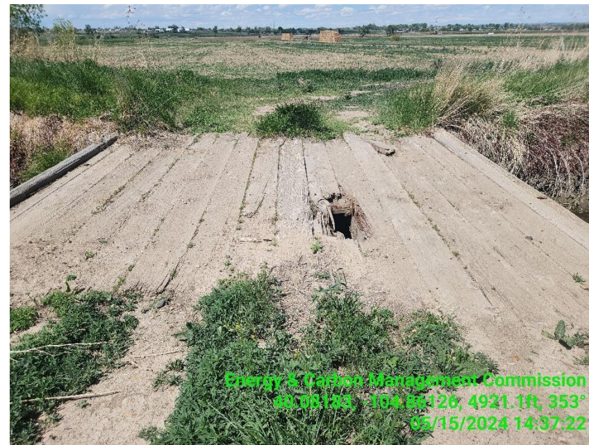
Photo 6 Access road bridge has damage on both ends and center decking.
