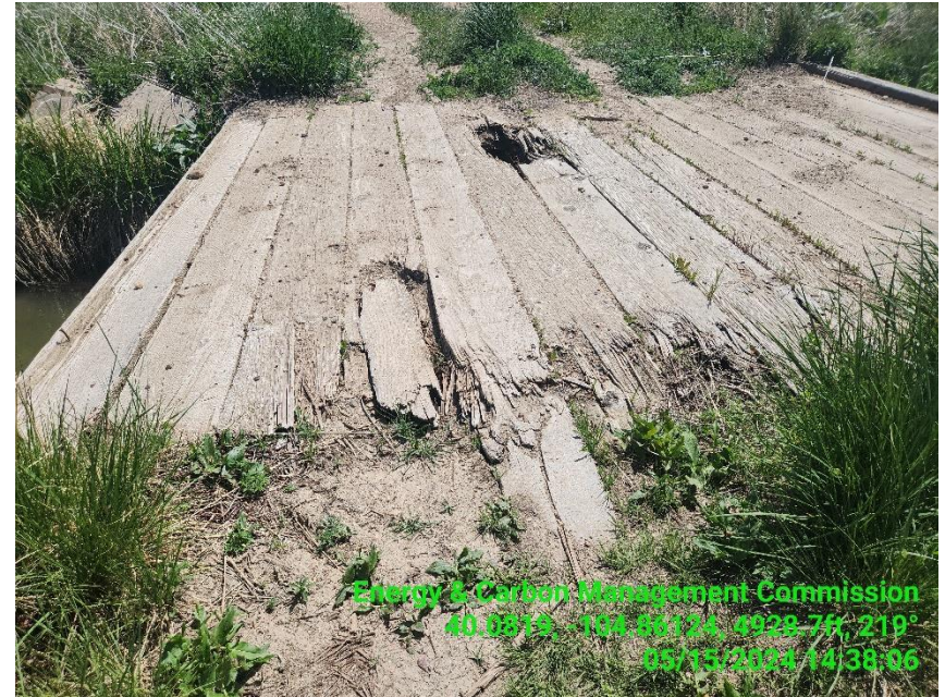
Photo 10 Access road bridge has damage on both ends and decking.
