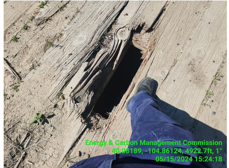
Photo 8 Access road bridge hole in decking Approx. 2.5 ft. x 1 ft.
