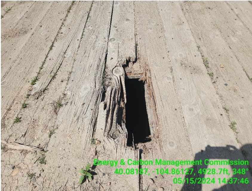
Photo 7 Access Road Bridge severe damage in the decking, irrigation water is visible below.
