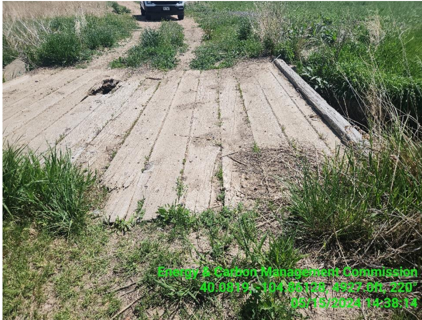
Photo 9 Access road bridge has damage on both ends and decking.
