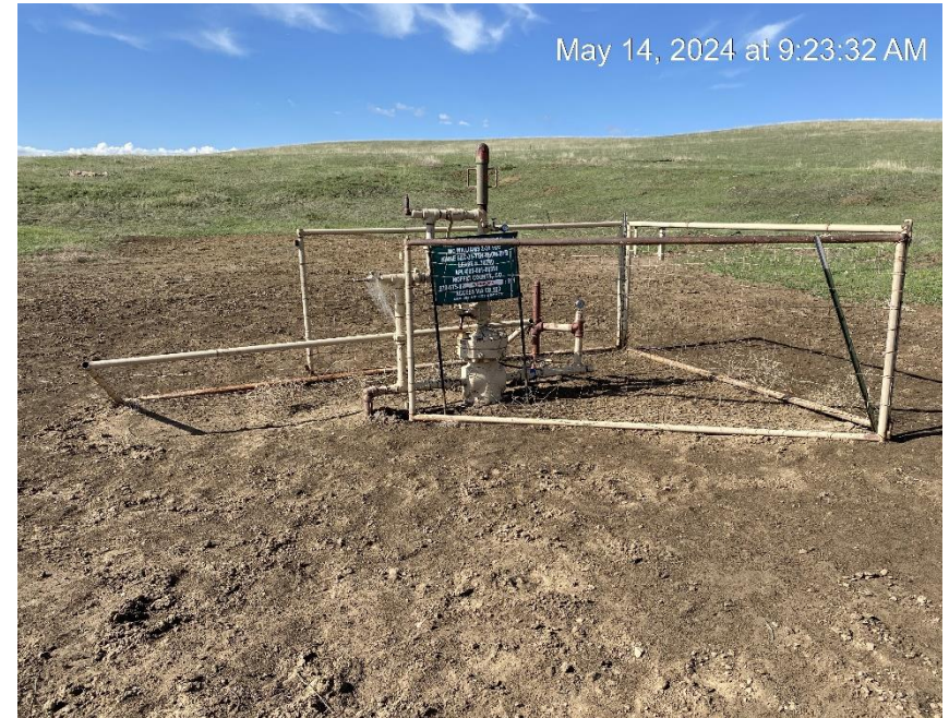
Wellhead fencing down. Possible wellhead leak
