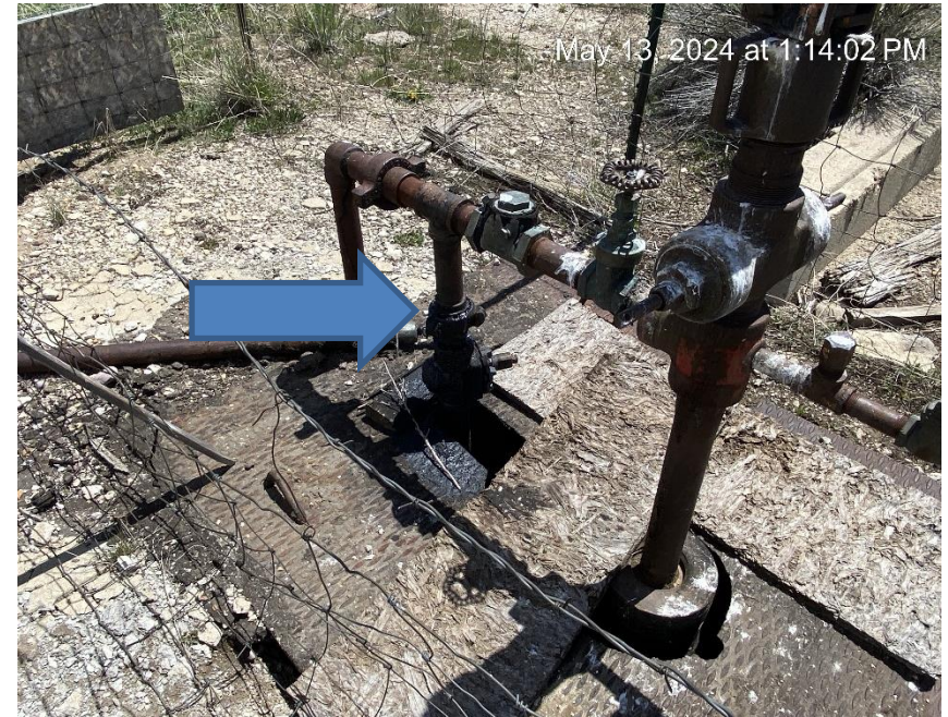
Flow line leak
