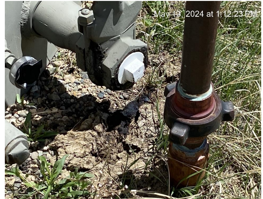
PVC cap leaking on tank valve
