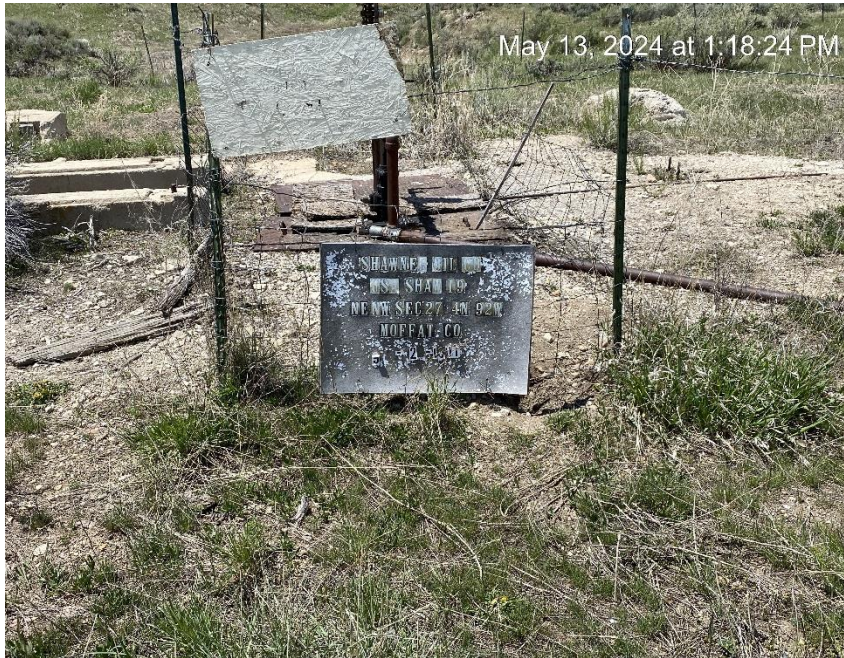
Wellhead sign missing required information
