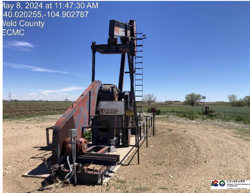
Pic 1 wellhead / pump jack
