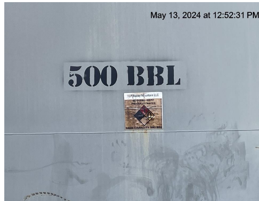
Photo # 6721 Tank label weathered & starting to become illegible.
