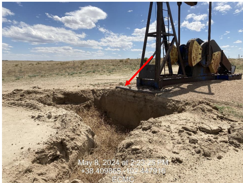
Photo 3 – Wellhead excavation
