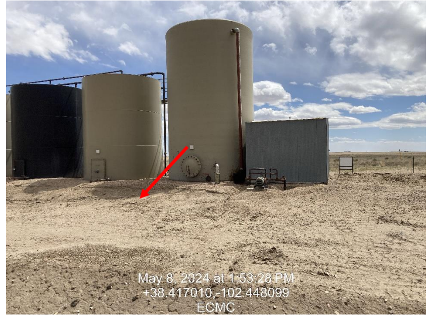
Photo 6 – Tank Battery, Open Excavation for Remediation # 34392
