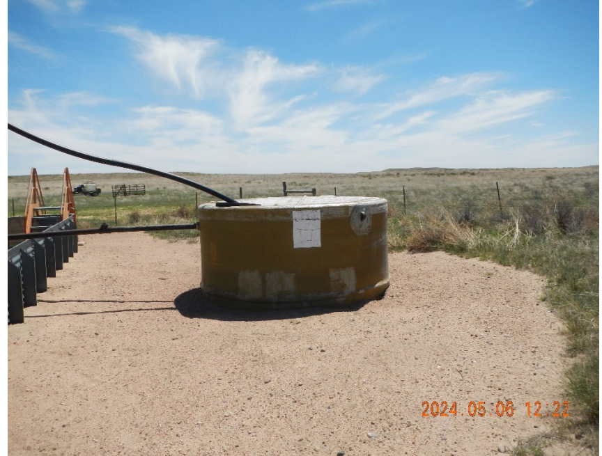
8. Partially buried over flow tank.
