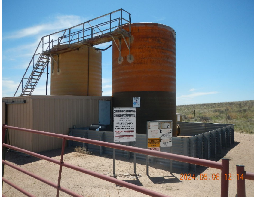
7. Battery AST tanks inside metal containment.
