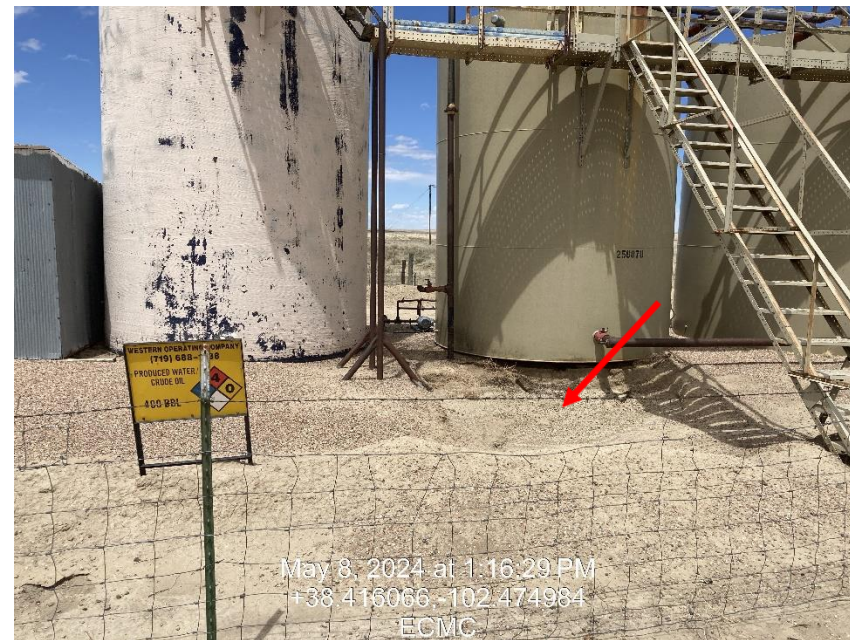
Photo 2 – Open Remediation excavation Impacted soils observed under tank
