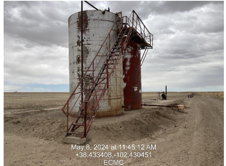
Photo 6 – Tank Battery, Secondary containment not adequate
