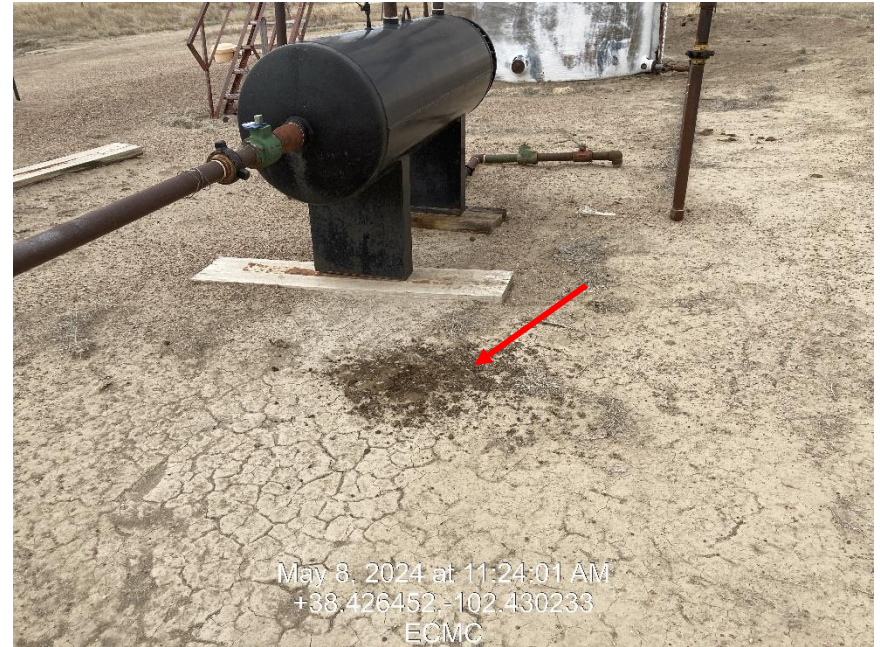
Photo 10 – Impacted soils in Secondary Containment
