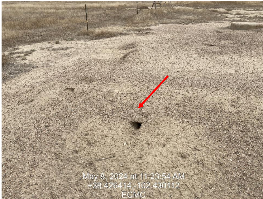
Photo 9 – Breach in Secondary Containment
