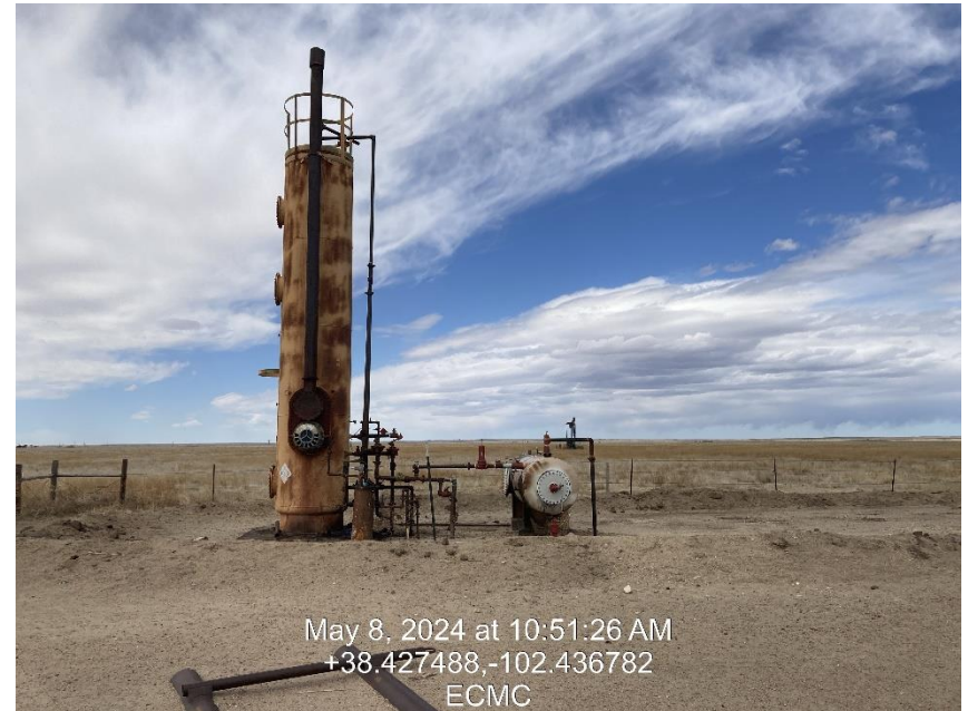
Photo 6 – Tank Battery / Treater
