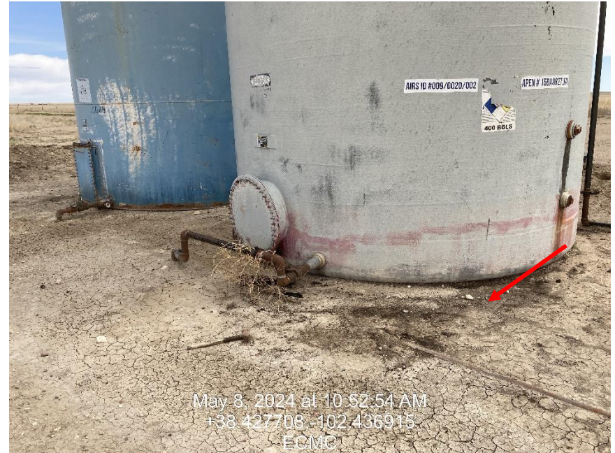
Photo 10 – Impacted soils in Secondary Containment
