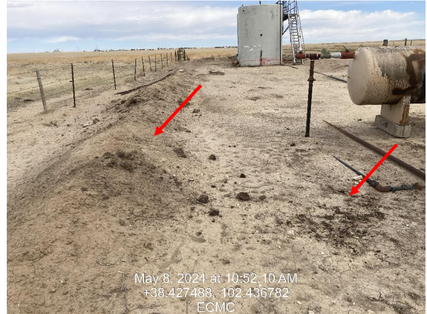
Photo 8 – Impacted soils in Secondary Containment
