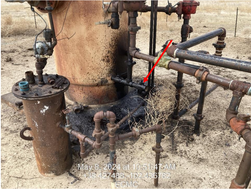
Photo 7 – Leaking piping at Treater.
