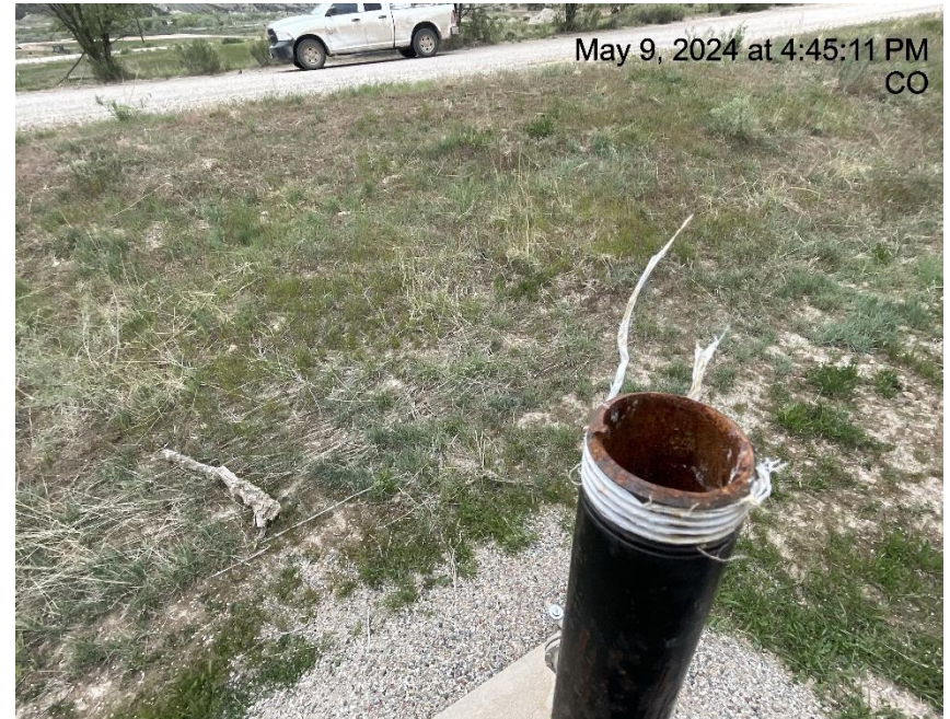
Photo # 6609 PRV vent line lacks cap/does not comply CECMC pressure safety device rules
