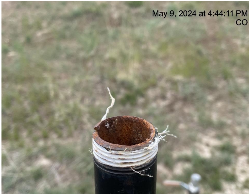
Photo # 6608 PRV vent line lacks cap/does not comply CECMC pressure safety device rules
