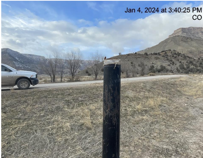
Photo # 1910 From inspection 708902696 conducted on 01/04/2024 PRV vent line lacks cap
