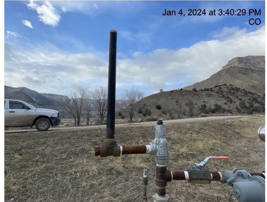
Photo # 1909 From inspection 708902696 conducted on 01/04/2024 PRV vent line lacks cap
