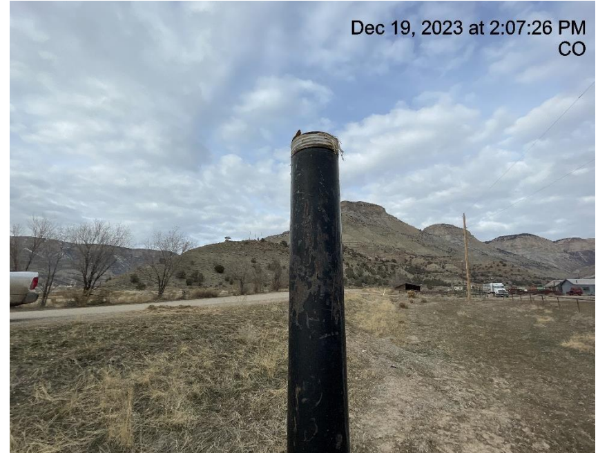
Photo # 385 From inspection 708902565 conducted on 12/19/2023 PRV vent line lacks cap
