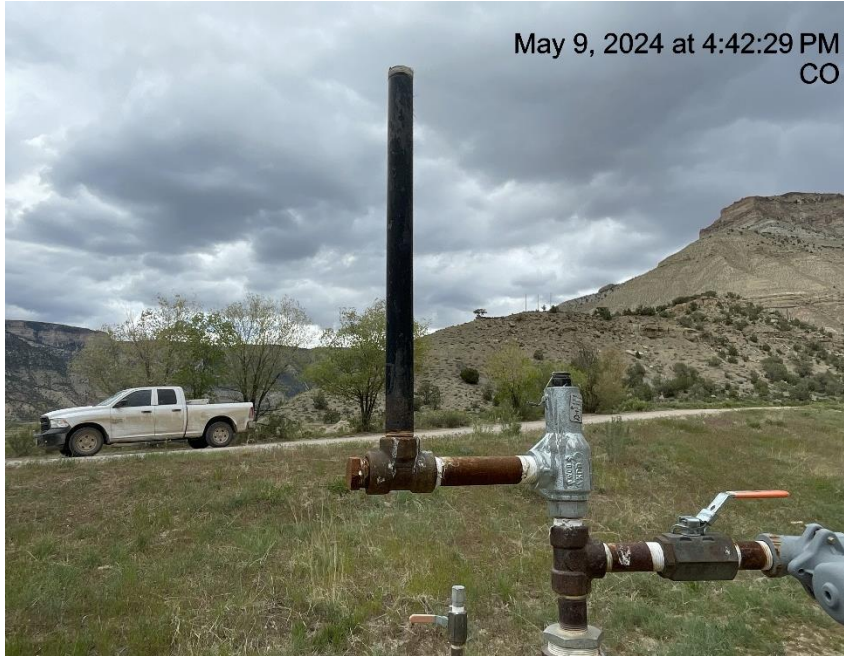
Photo # 6606 PRV vent line lacks cap/does not comply CECMC pressure safety device rules
