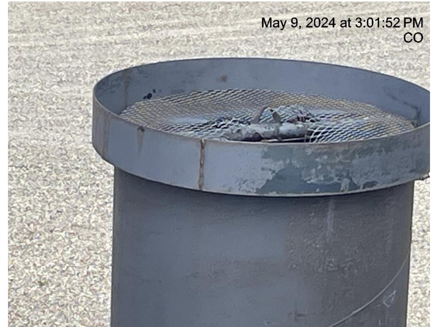
Photo # 6537 Bird protection on ECD damaged & needs maintenance/wildlife hazard/available for entry by wildlife
