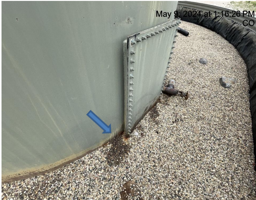
Photo # 6456 Suspected tank leak/tank appears to lack integrity (Tank # 81735)
