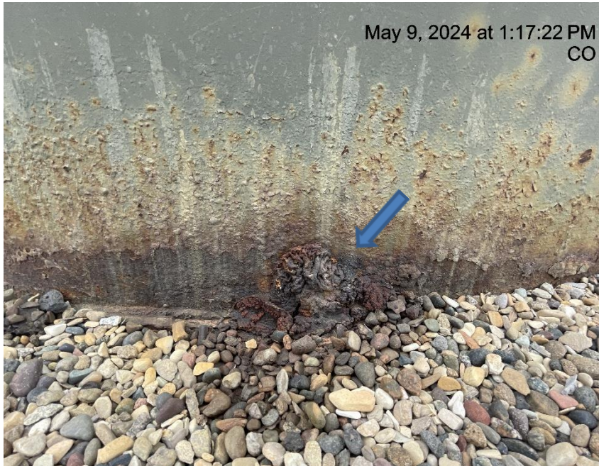
Photo # 6458 Suspected tank leak/tank appears to lack integrity (Tank # 81735)
