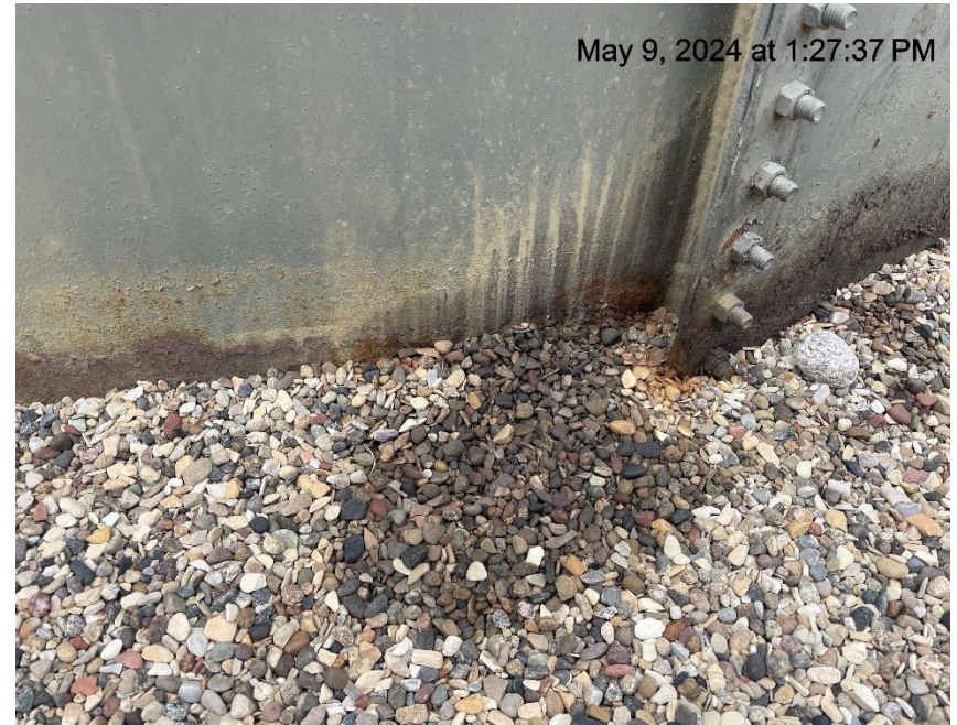
Photo # 6457 Suspected tank leak/tank appears to lack integrity (Tank # 81735)
