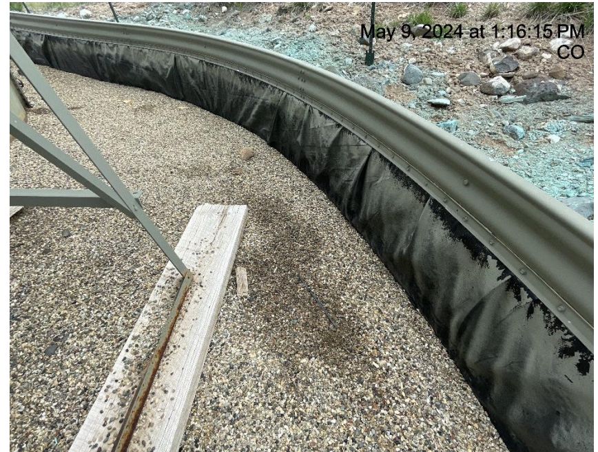
Photo # 6459 Stained gravel in secondary containment
