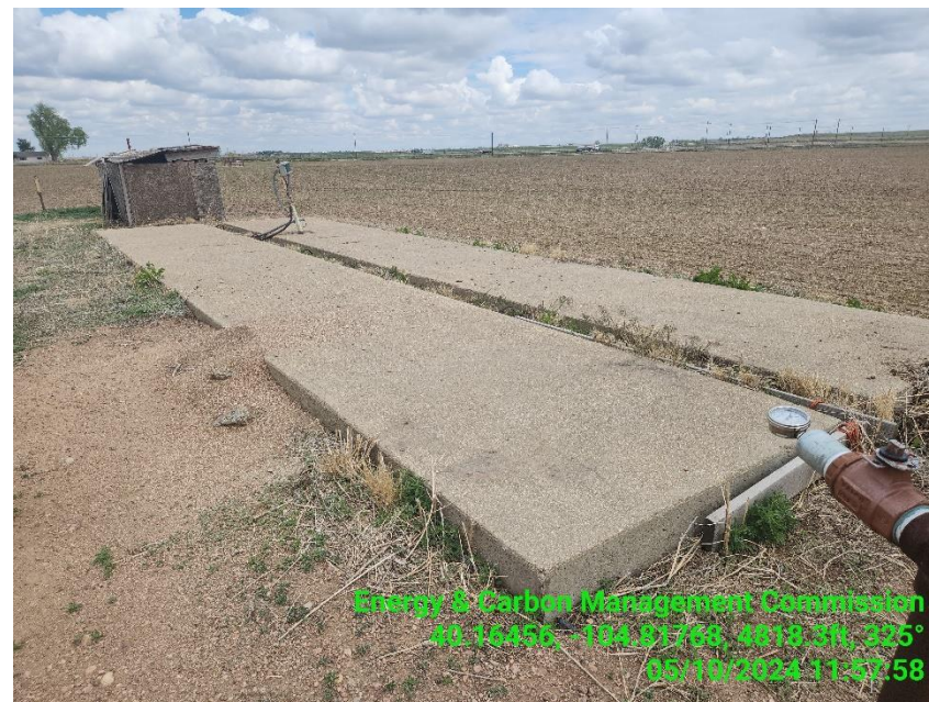
Photo 4 Unnecessary equipment, old pump jack base.
