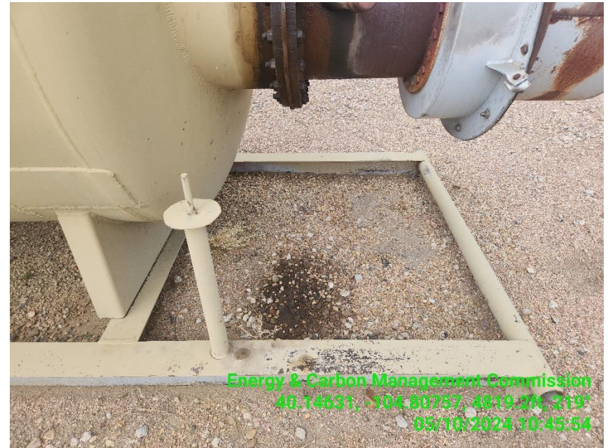
Photo 8 HHT leak dripping onto the ground.
