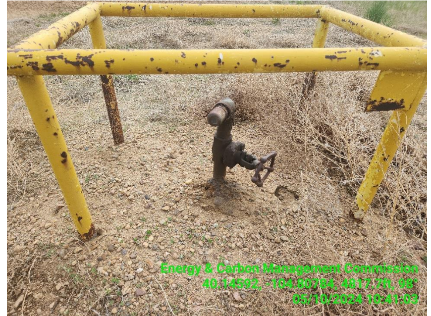
Photo 12 Stained soil around flow line riser west of the TB.
