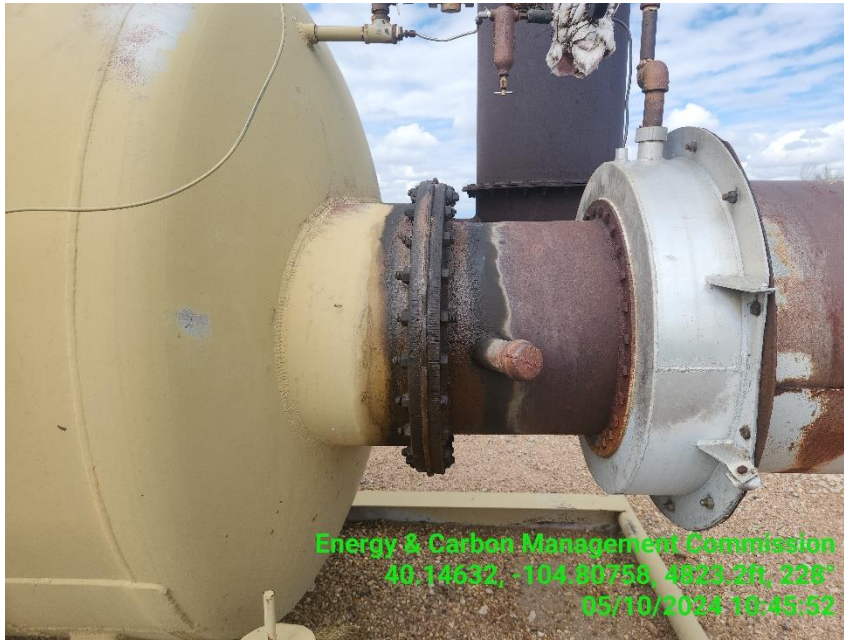
Photo 7 HHT gasket slowly leaking.
