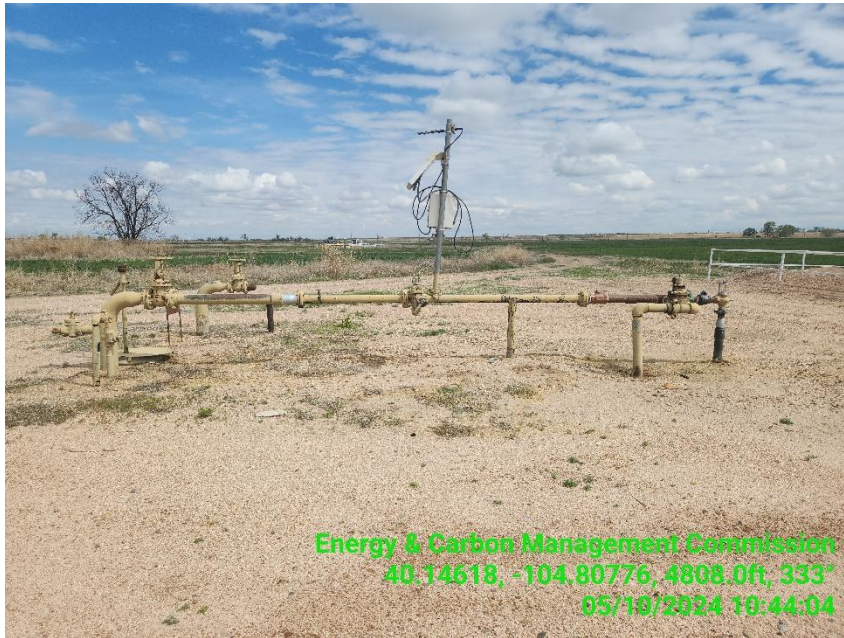
Photo 5 Gas Meter Run.
