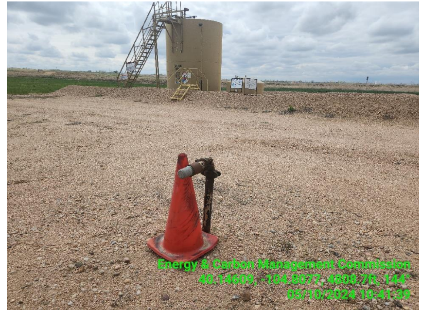
Photo 14 Flow line riser.
