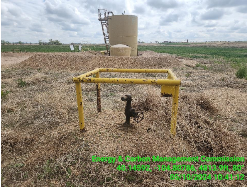
Photo 11 Stained soil around flow line riser west of the TB.
