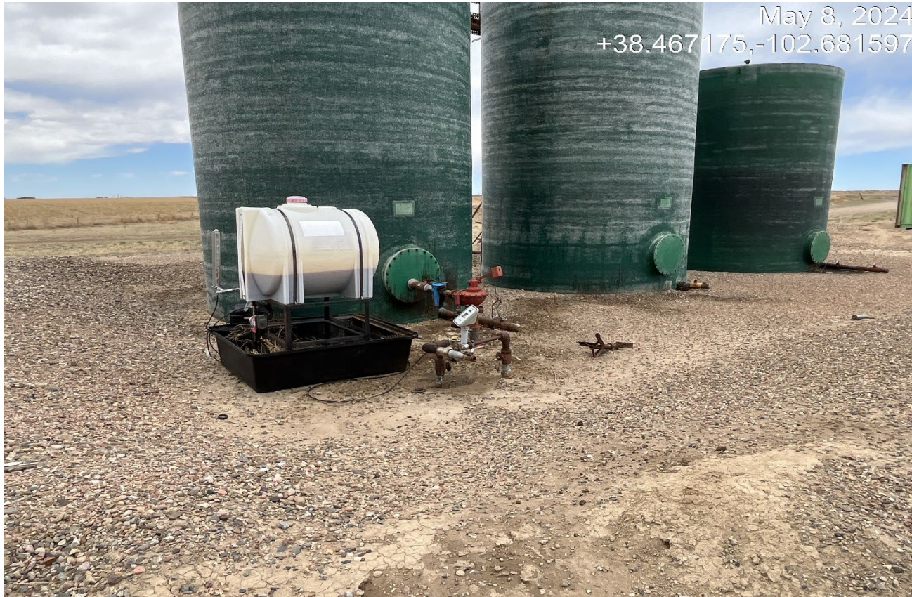
Photo 7. There are stained soils at the back side of the tank battery that must be cleaned up.
