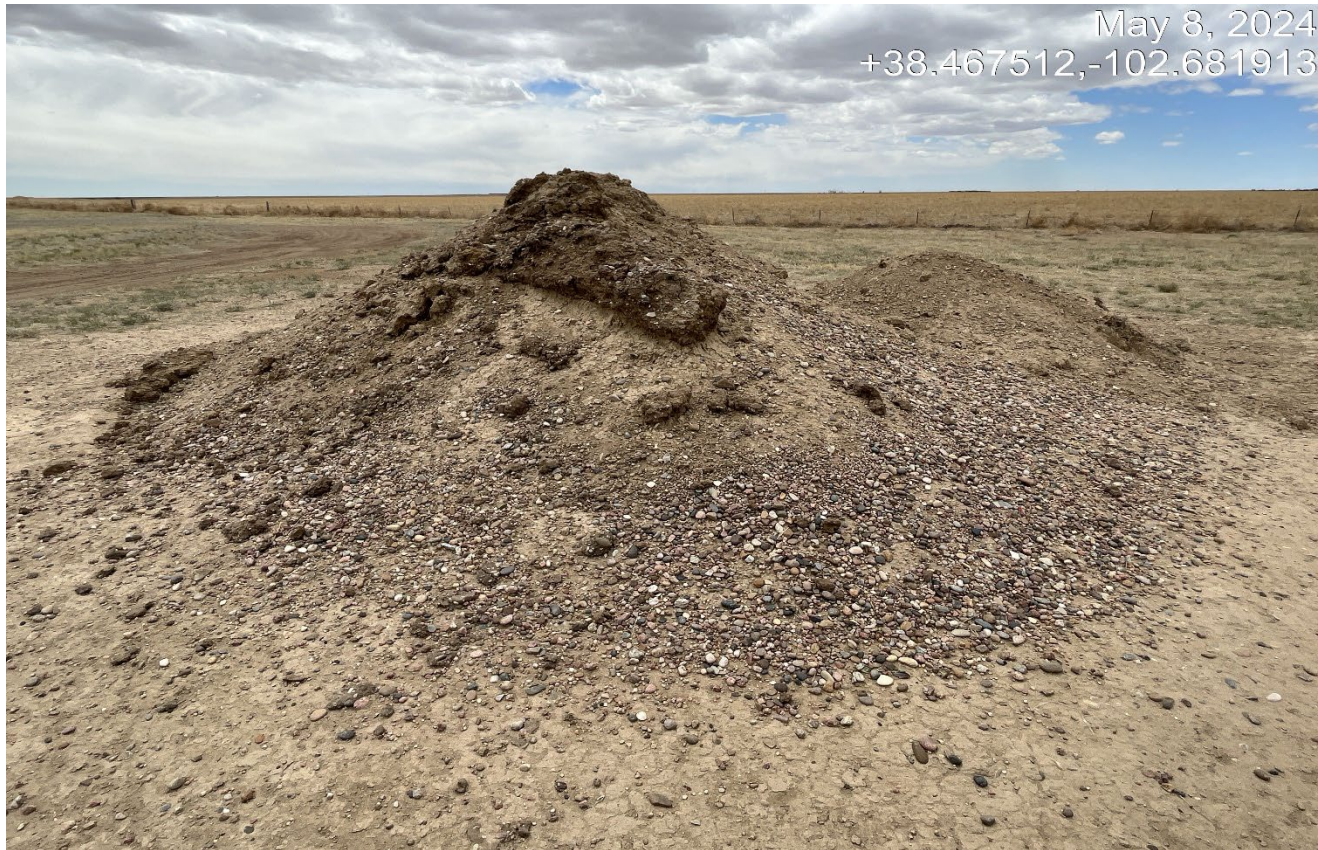
Photo 2. There is a pile of oily gravel material stored on location that must be removed and properly disposed.
