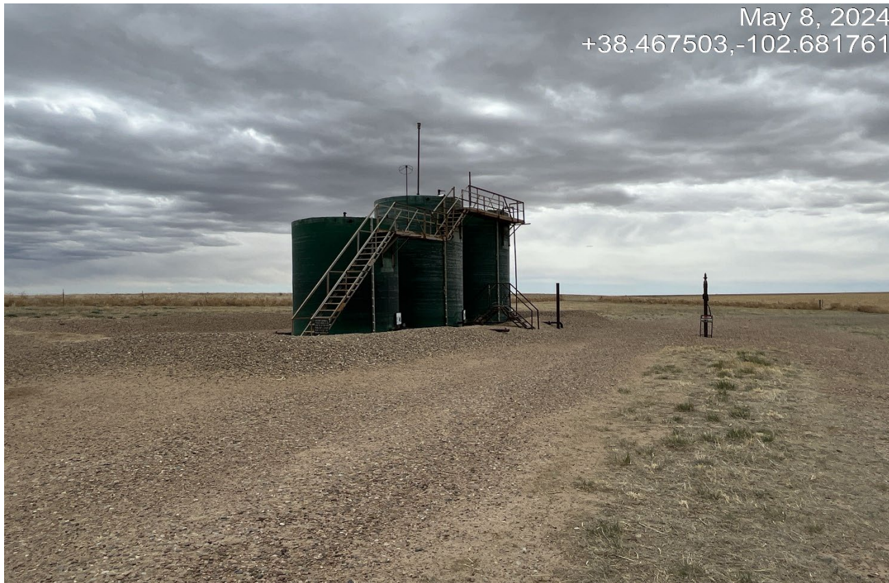
Photo 6. Facing toward the tank battery. The H2S wind sock is missing.
