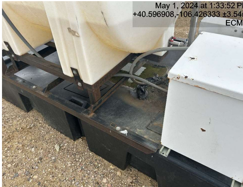
Chemical tank containment is full of fluid
