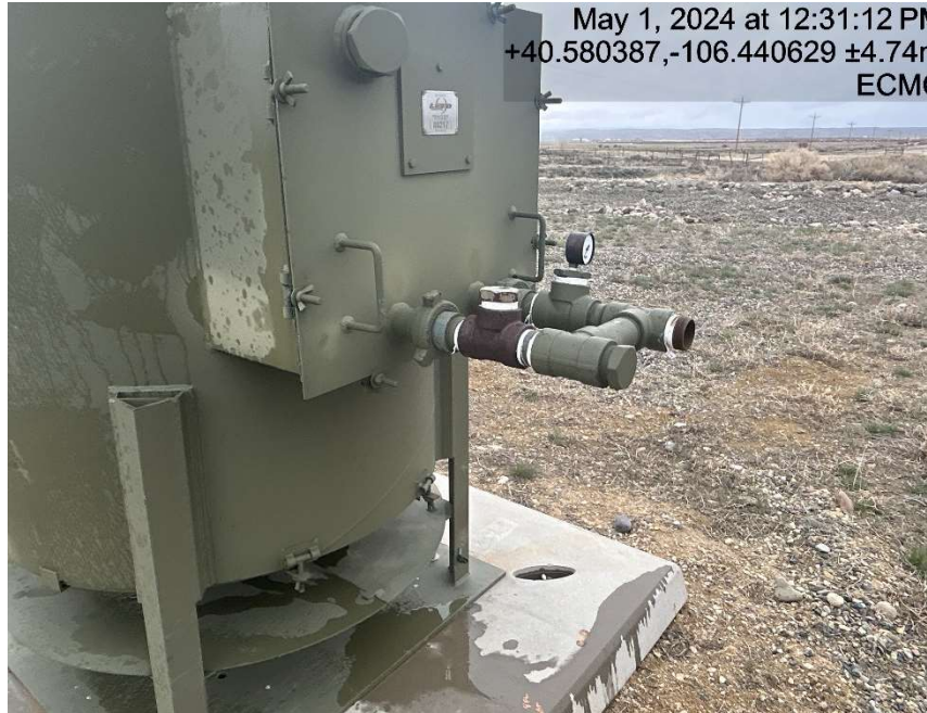
ECD is disconnected and open hole for wildlife to enter
