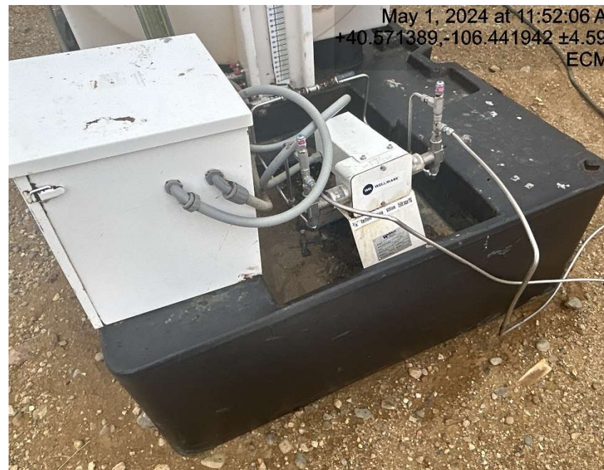
Chemical containment is full of fluid
