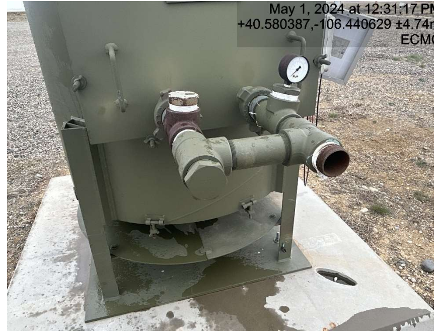
ECD is disconnected and open hole for wildlife to enter
