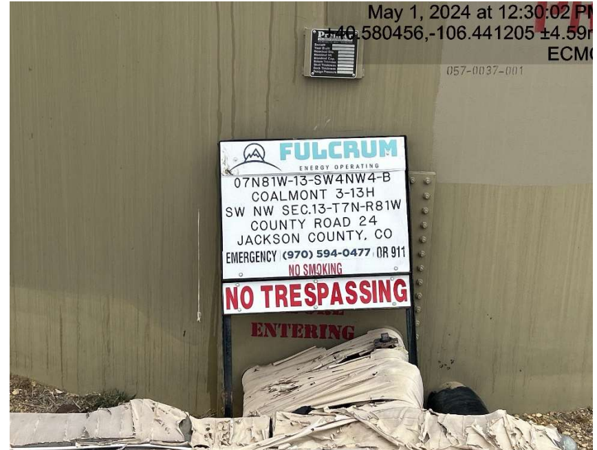
Battery signage lacks API
