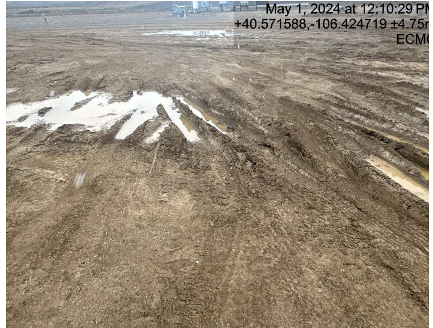
Lack of stabilization/compaction
