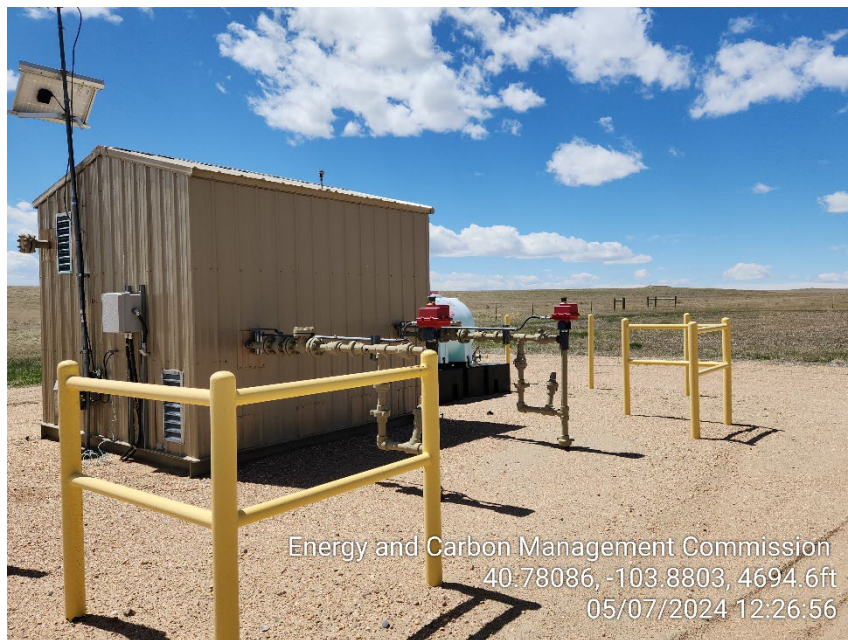
Photo 1 – Gas Lift Injection Meter Houses
