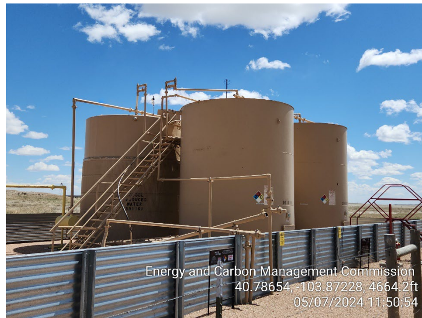
Photo 2 – Tank Battery
