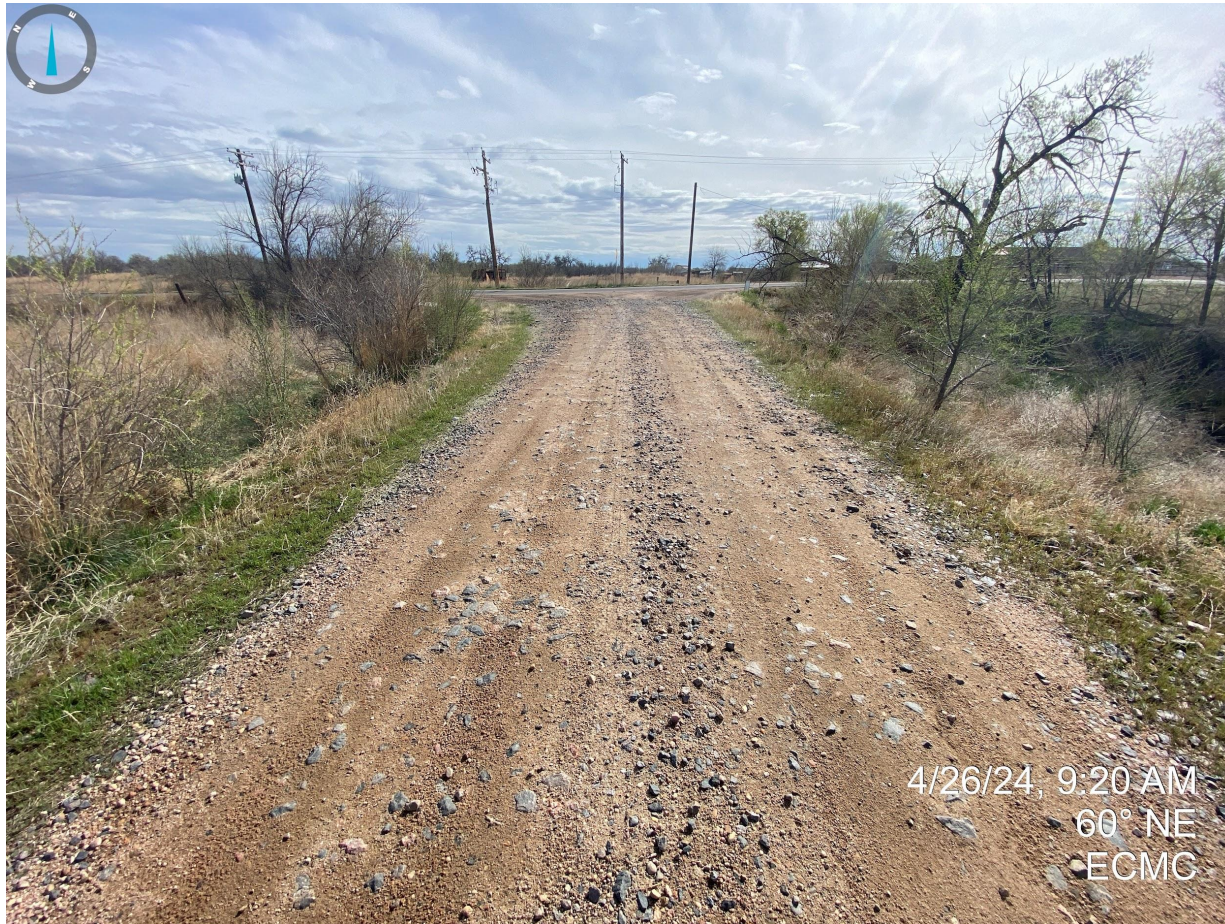
Photo 11. Vehicle track out pad requires maintenance.
