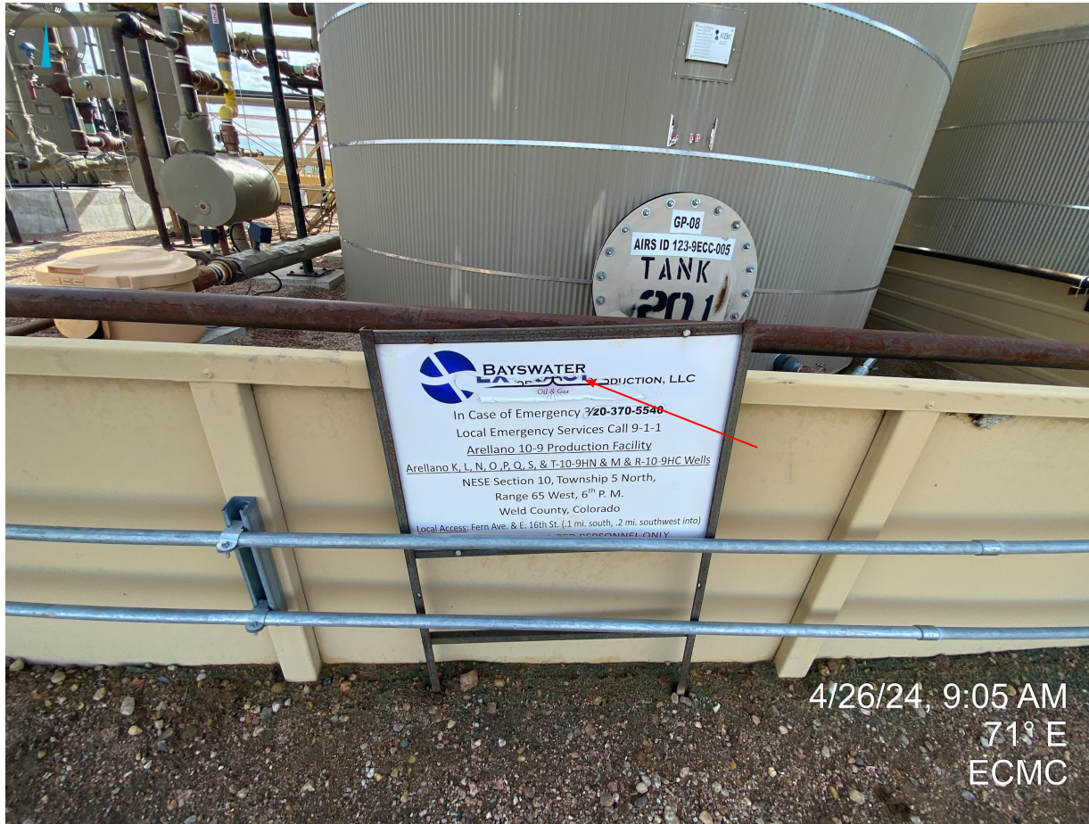
Photo 17. Sign at tank battery is peeling, faded, cracked.
