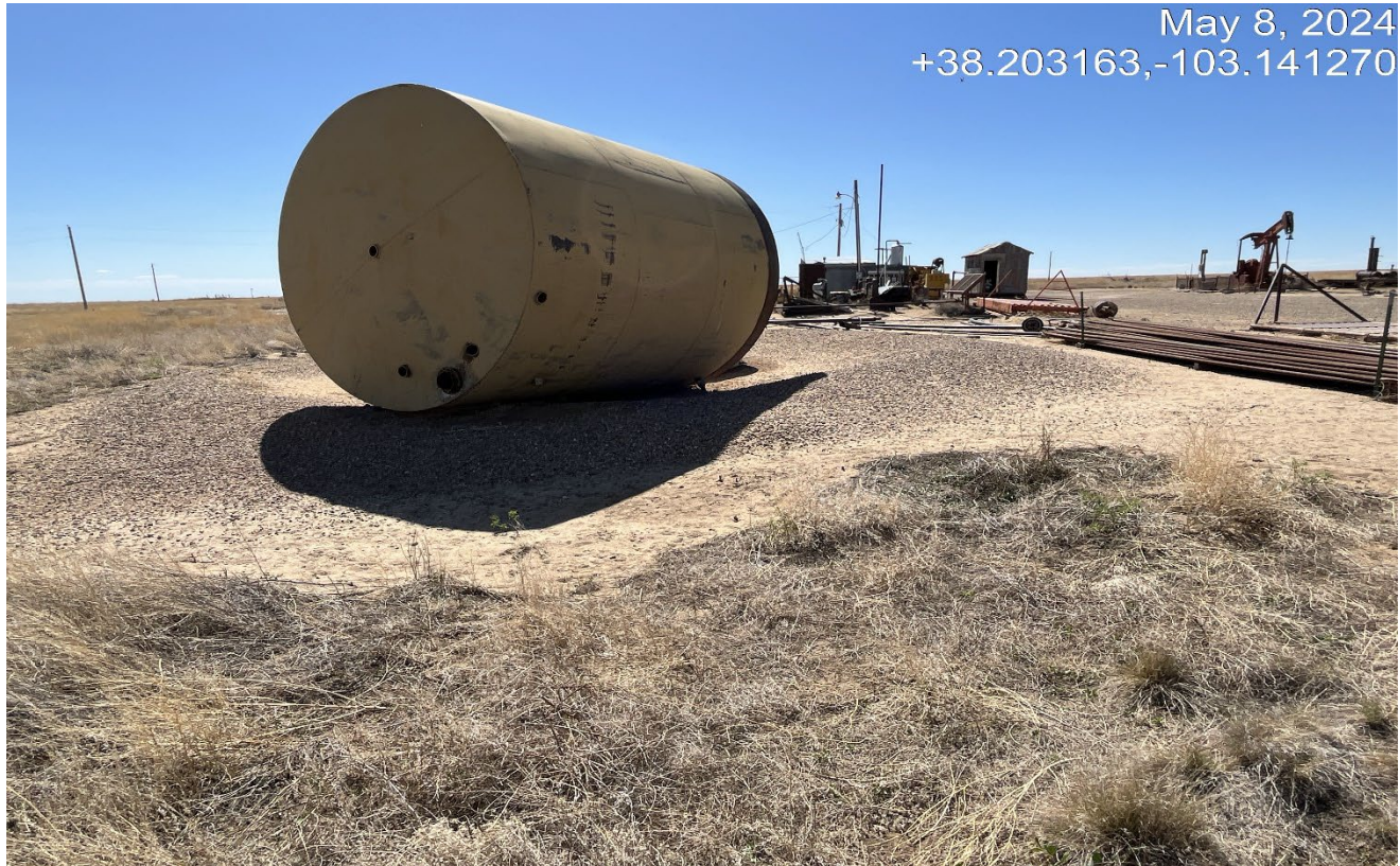
Photo 21. East side of the location facing west. There is unused pipe stored on location and a tank that is tipped over.
