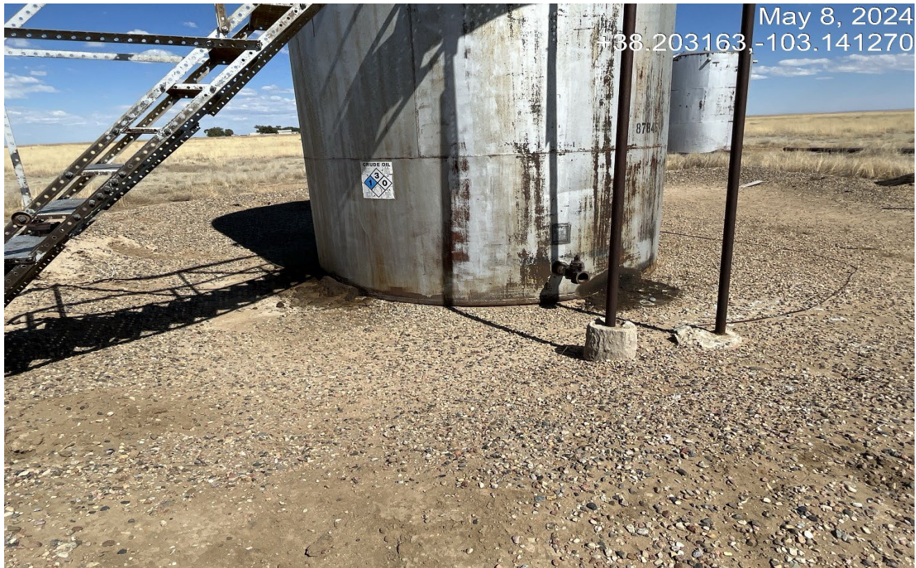
Photo 20. There is oily sludge at the base of the tank that needs to be cleaned up and properly disposed.
