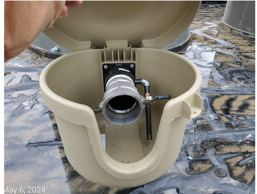
Photo 6: Photo examples showing lines at tanks missing cap/plug.
