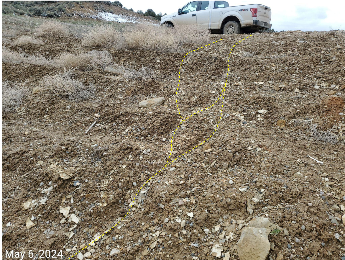
Photo 12: Continued from photo 11. Photo taken down slope of the working pad surface, facing west. Slopes bare and lack BMPs to stabilize, as well as to minimize erosion and degradation.
