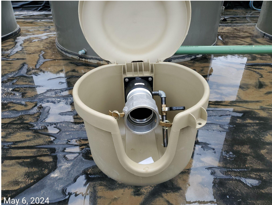
Photo 6: Photo examples showing lines at tanks missing cap/plug.
