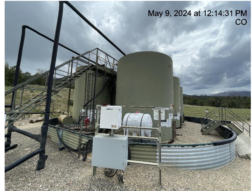
Photo # 6383 Tank battery lacks required signage
