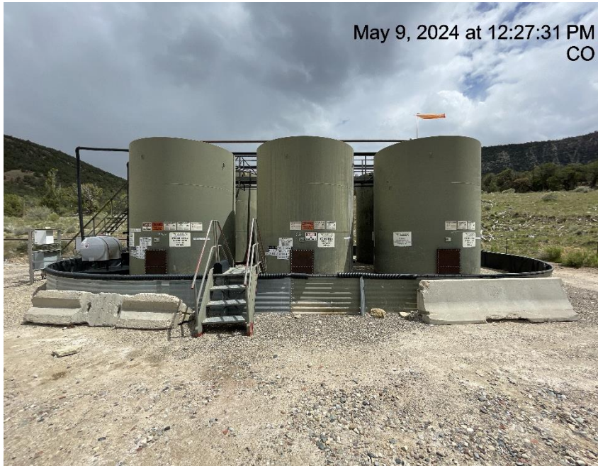
Photo # 6380 Tank battery lacks required signage
