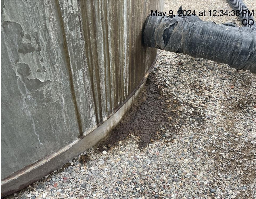
Photo # 6386 Stained gravel in secondary containment
