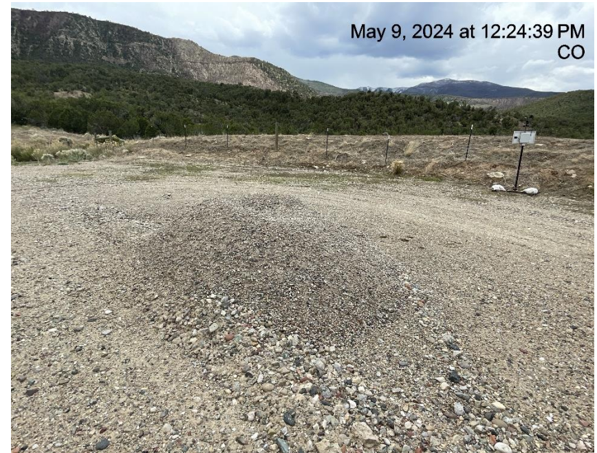
Photo # 6388 Stockpiled soils with no BMP's
