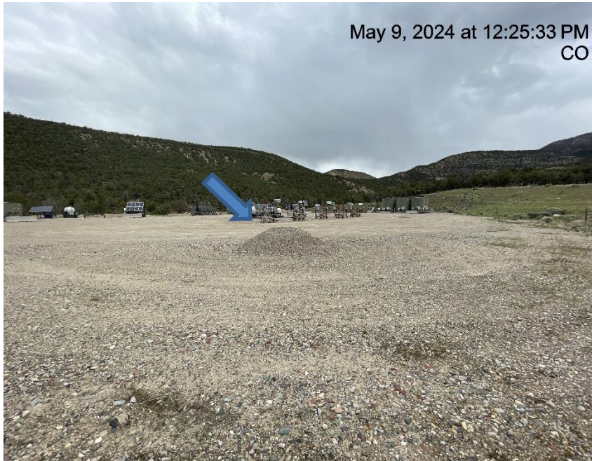
Photo # 6387 Stockpiled soils with no BMP's
