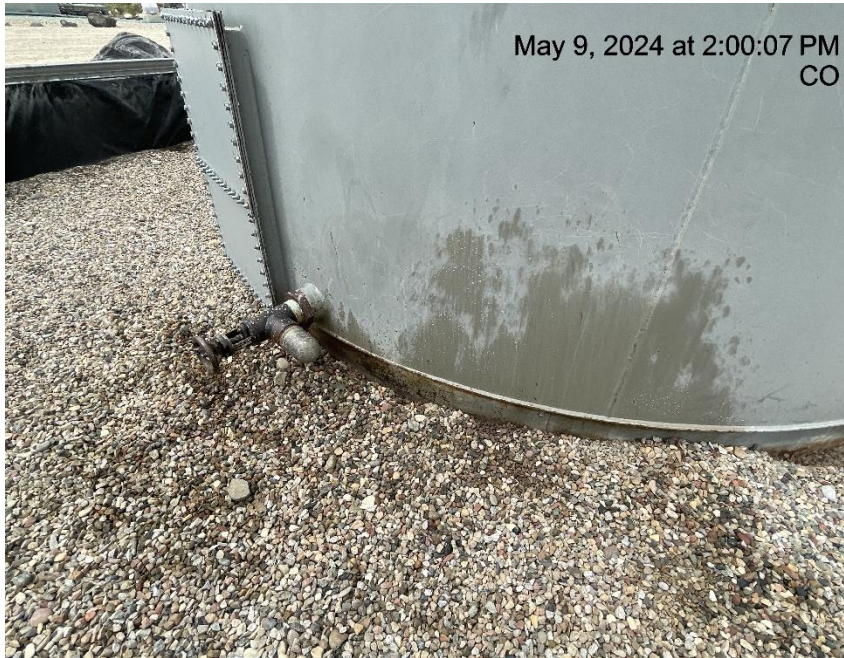
Photo # 6499 Stained gravel in secondary containment
