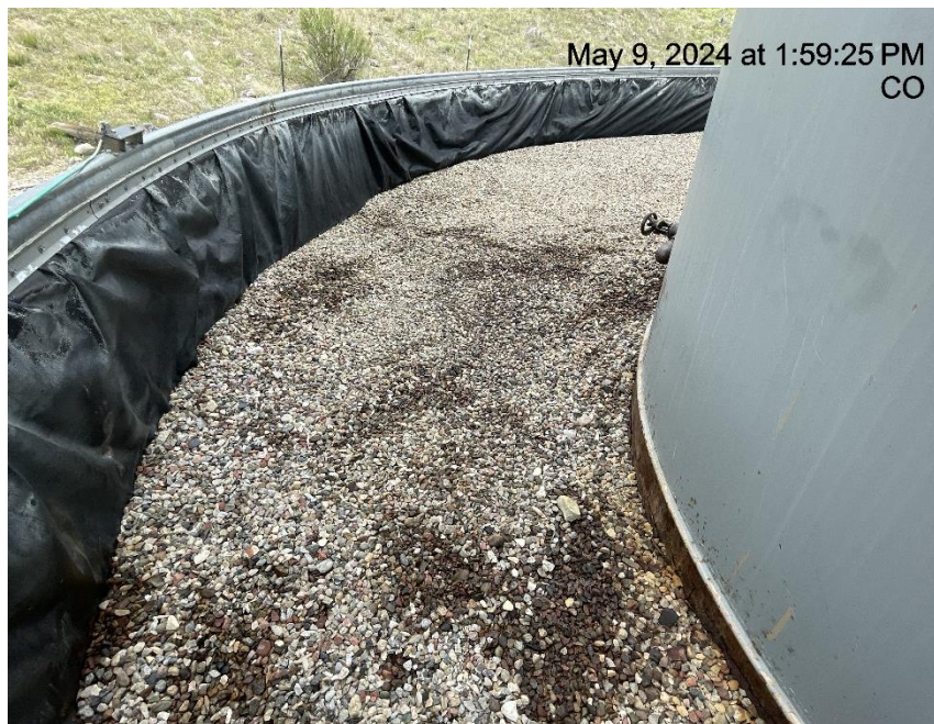
Photo # 6497 Stained gravel in secondary containment
