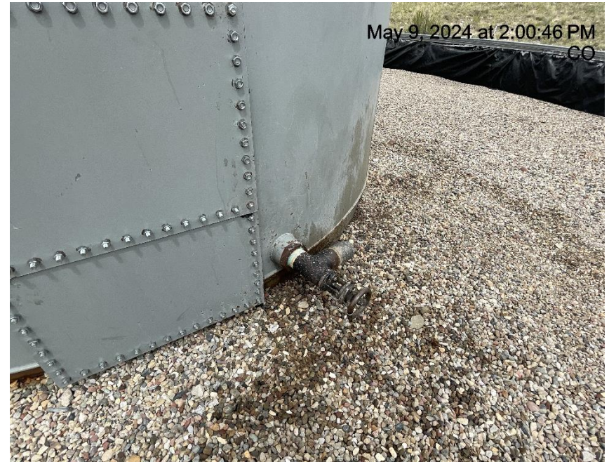
Photo # 6500 Stained gravel in secondary containment
