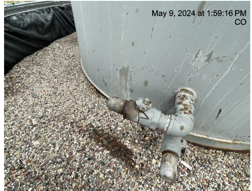
Photo # 6496 Stained gravel in secondary containment
