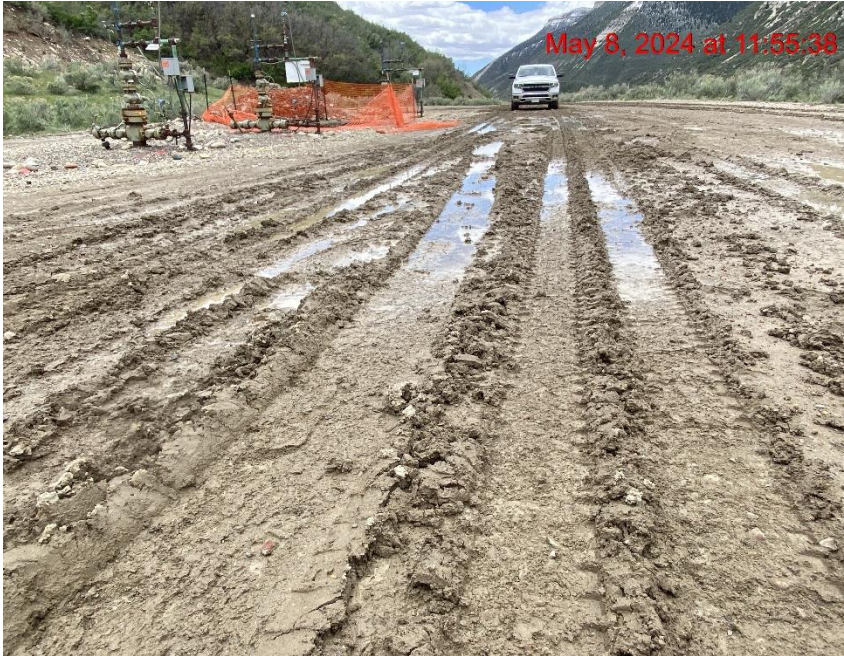
Lack of Stabilization – Photo #01008
