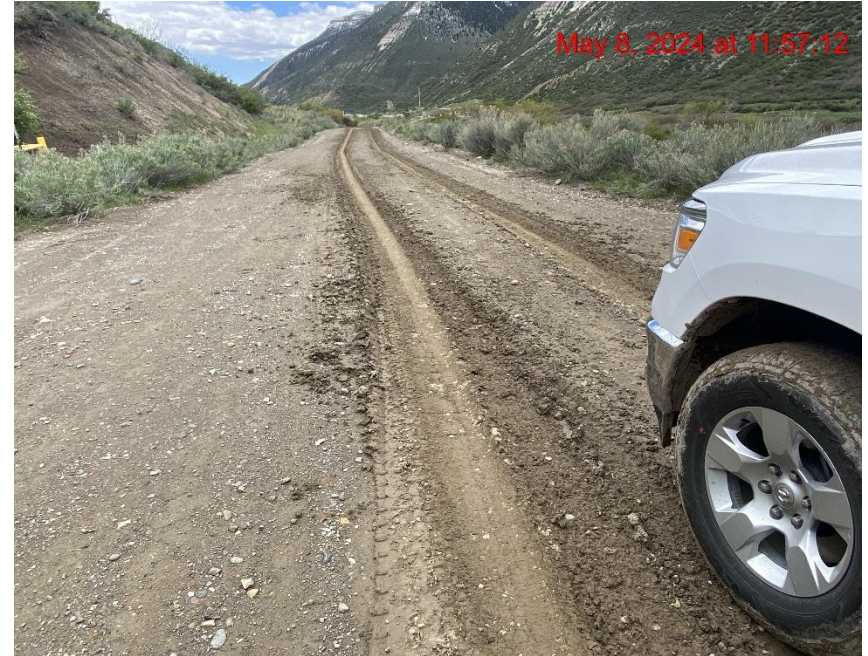
Insufficient Vehicle Tracking BMPs at Location Entrance/Exit – Photo #01009
